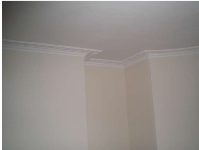
Cornice to first floor front room 196 Parrock Street
