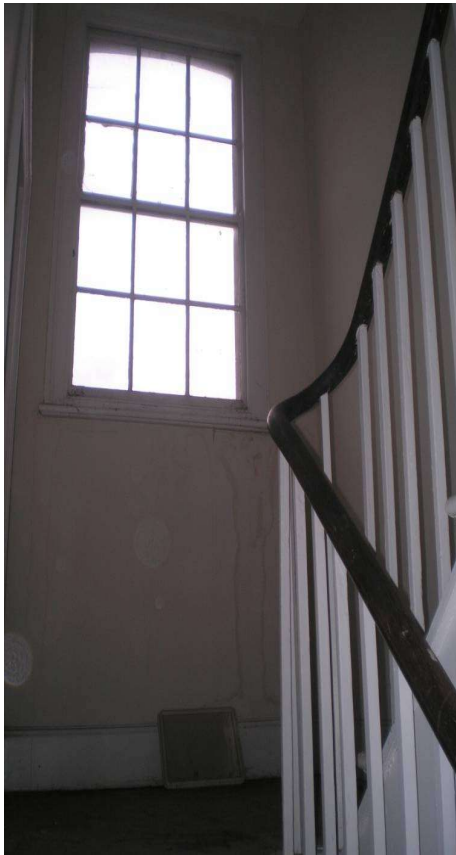
Bannister between ground and first floors
