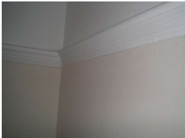
Picture rail in first floor rear room 196 Parrock Street
