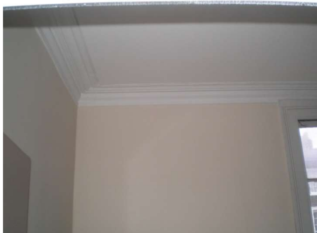
Cornice to first floor front room 197 Parrock Street
