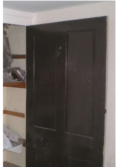
Cupboard door in 3 rd Floor front room Original frame visible
