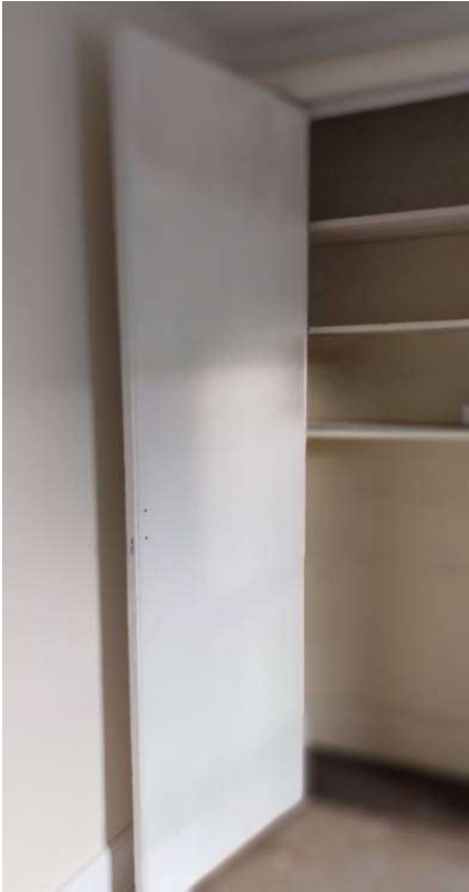
Cupboard door in 1 st floor rear room 197 Parrock Street Original frame not visible
