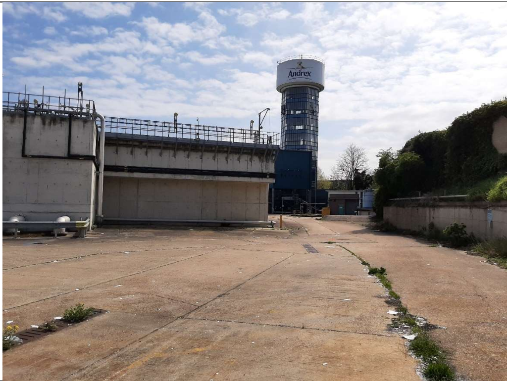
4. Effluent Treatment Plant and Water Tower.
