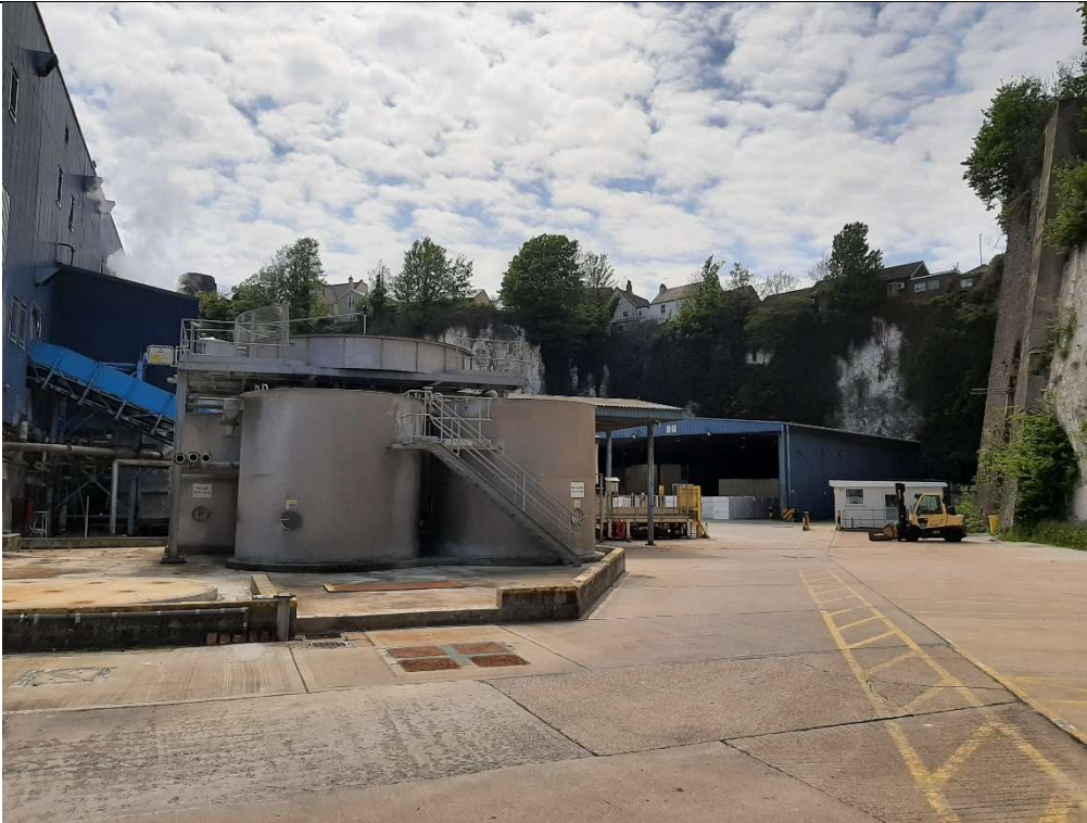
7. Storage tanks in southern area looking SE.
