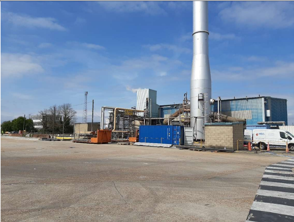
1. Boiler House Looking NW.
