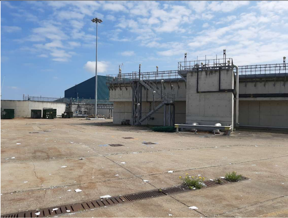
5. Effluent Treatment Plant Looking E.
