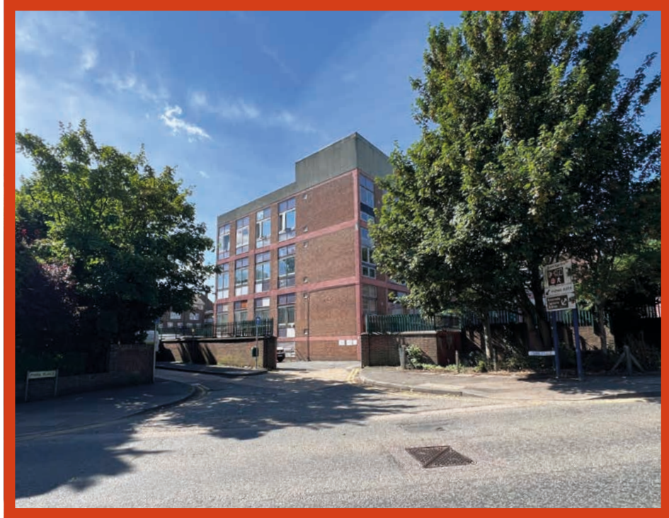
Telephone Exchange - View South from Ordnance Road
