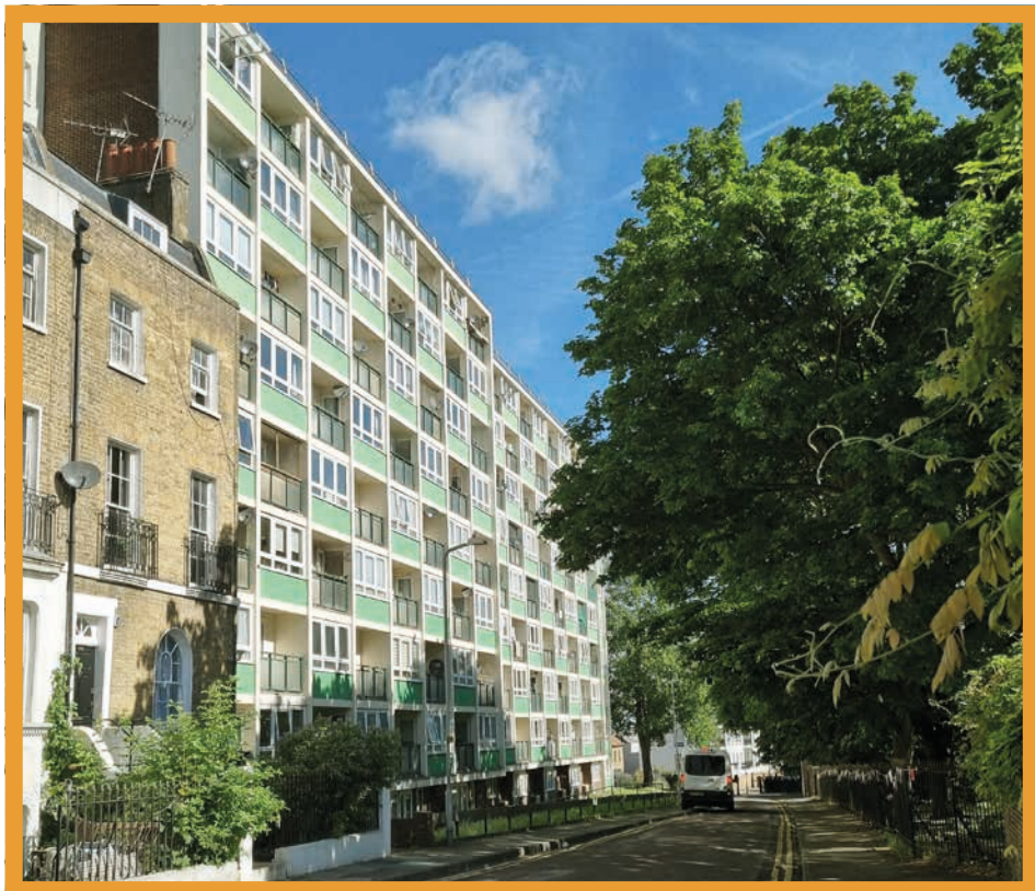
View North along Milton Place
