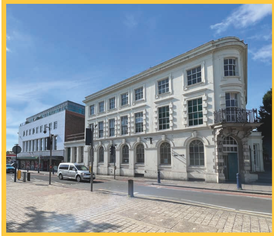
Berkley Crescent & The Grove Junction
