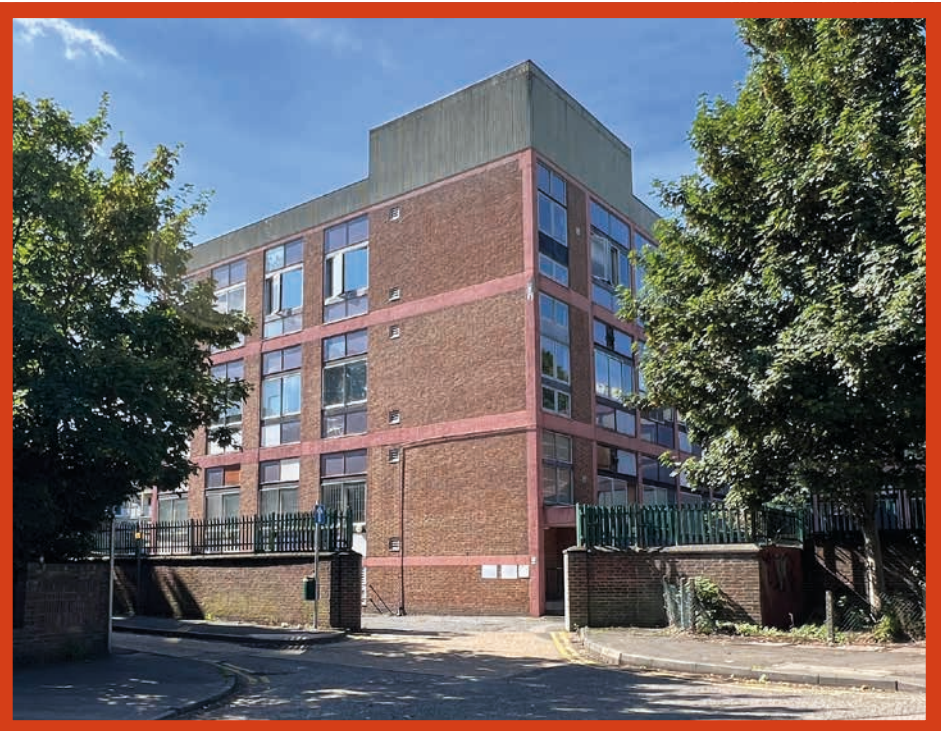
Telephone Exchange - View South from Ordnance Road
