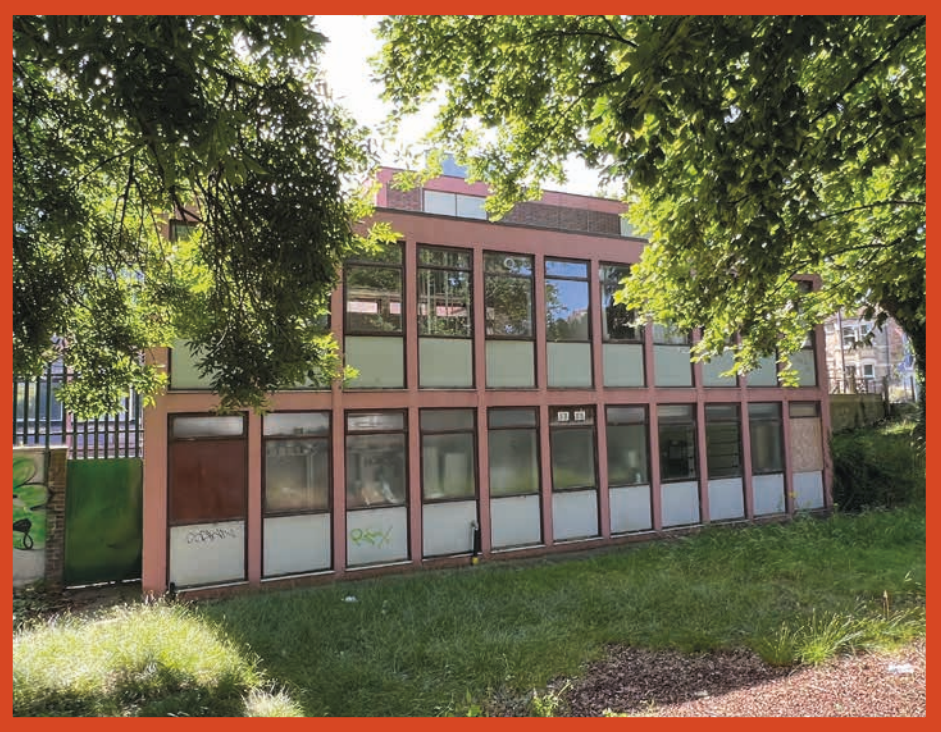
Telephone Exchange - View West from from Ordnance Road
