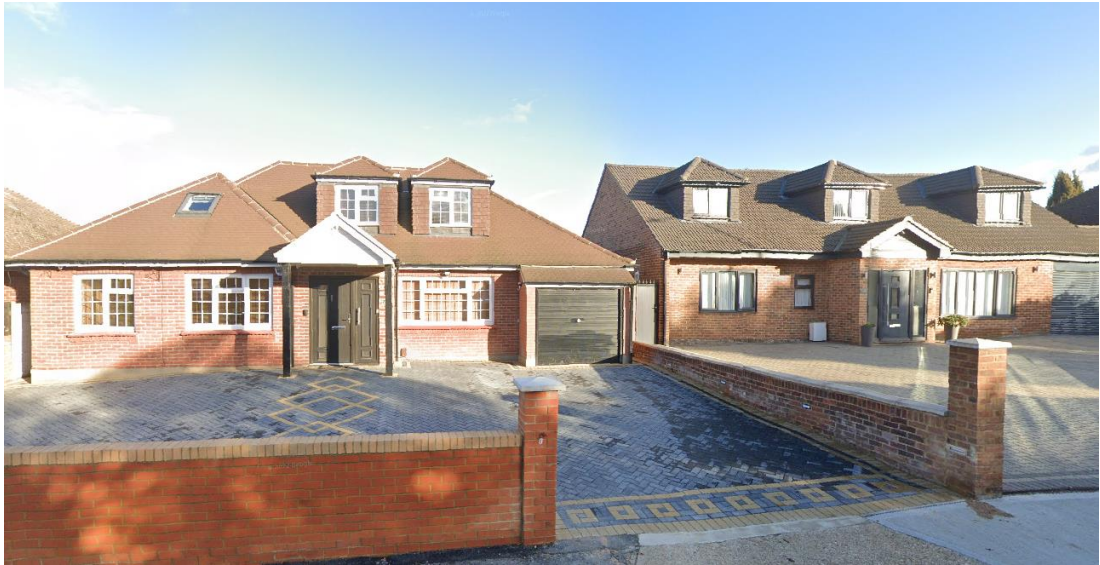
Nos. 224 and 226 Singlewell Road
