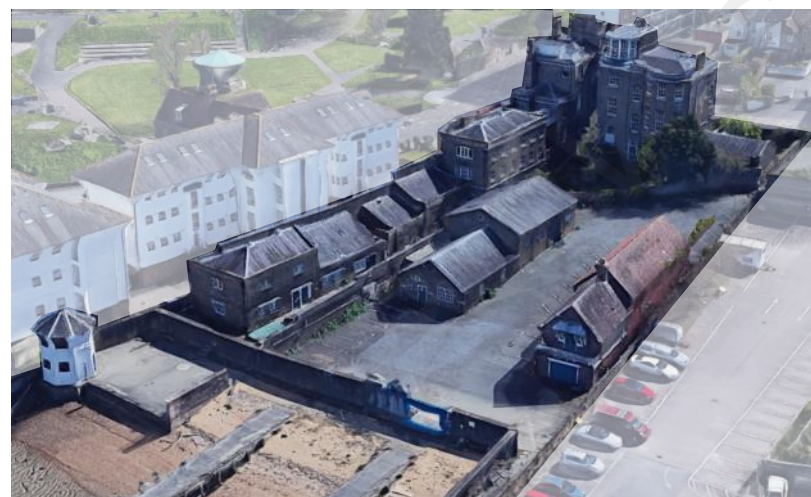
Aerial photograph of existing site as viewed from the north
