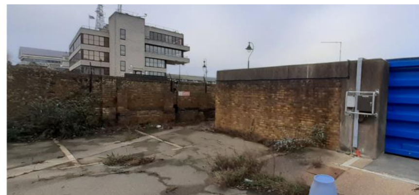
Photograph of Flood defence wall with PLA building visible behind.
