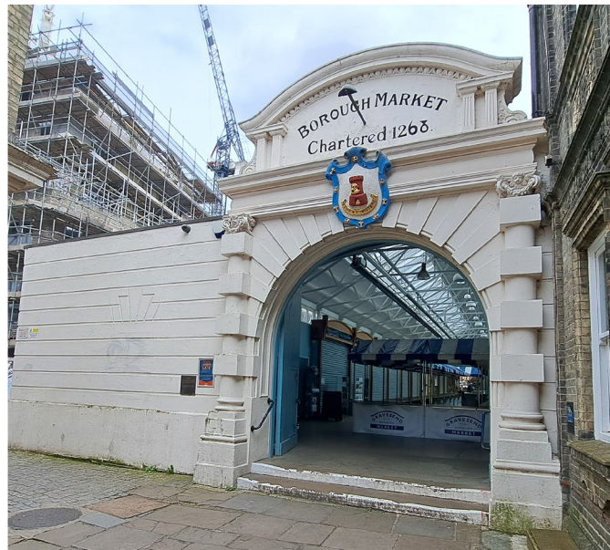
Existing Western Entrance
