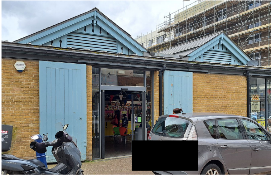
Existing Eastern Entrance
