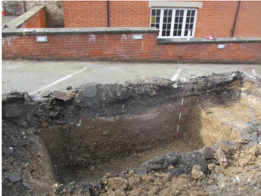
Plate 21. Trench 5, cut on a north-west-north/south-east-south alignment in the courtyard area west of the modern work shop area, exposed made ground with a maximum depth of 1.90m present here as a result of ground re-instatement following the construction of the sunken red-brick building shown in the background. The original excavation cut into alluvial clay-silt can be seen in the left part of the trench brickearth to the south. The made ground here was not evident in the opposite section (see Plate below) (1.4m scale)
