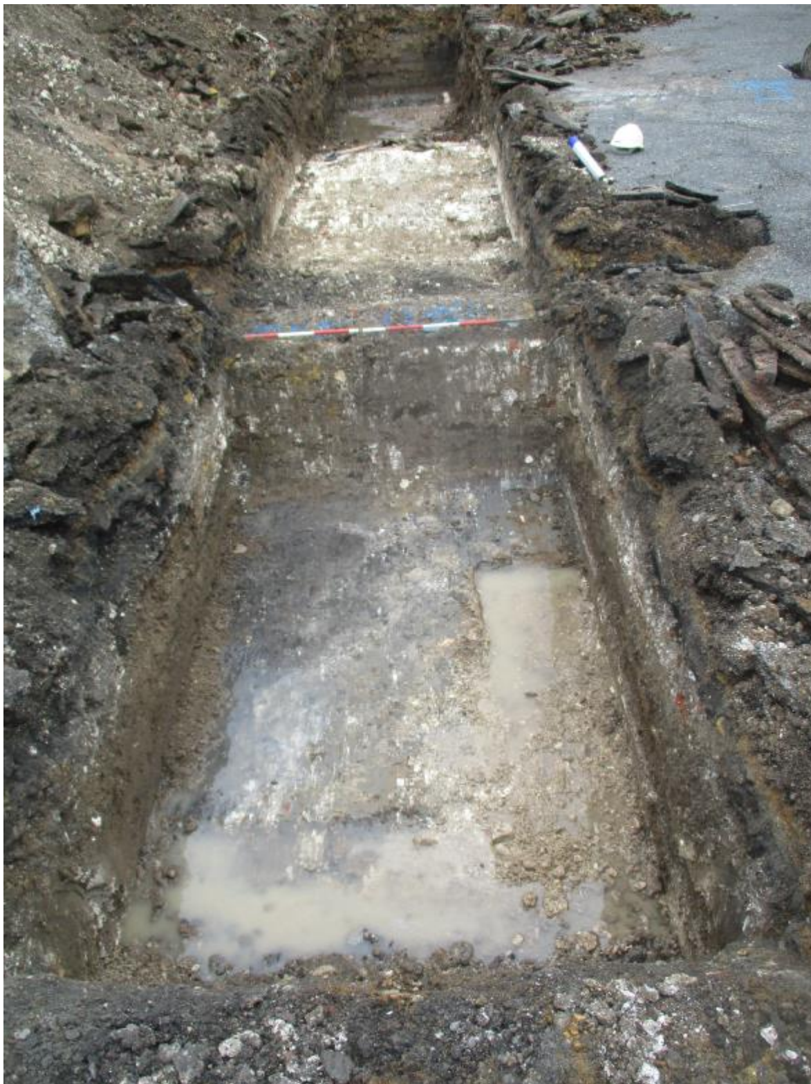
Plate 8. Trench 1 (east-west aligned in the northern part of the site) looking west with a 1.5m deep channel exposed in the background (assumed to provide access by boat to the boathouse shown in Plates 3, 4 & 6, a chalk floor in the mid-ground and two earlier channels in the back- and foreground (1.6m scale lying north-south over a still-functioning modern water main)
