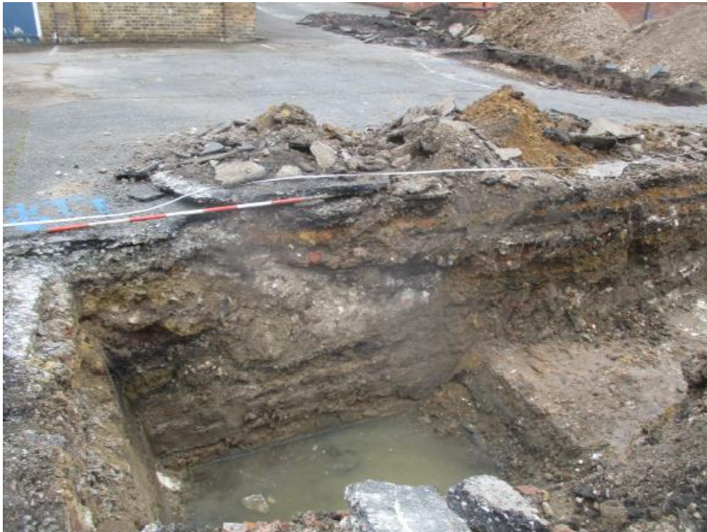
Plate 9. The eastern end of Trench 1 looking south showing the latest water channel (Channel 117, on the left/west) cutting an earlier channel capped by levelling deposits to the right, which cut a chalk layer/floor (114) adjacent to and was contemporary with the earliest exposed channel in the trench's west end. The boathouse can be seen in the background (1.4m scale)
