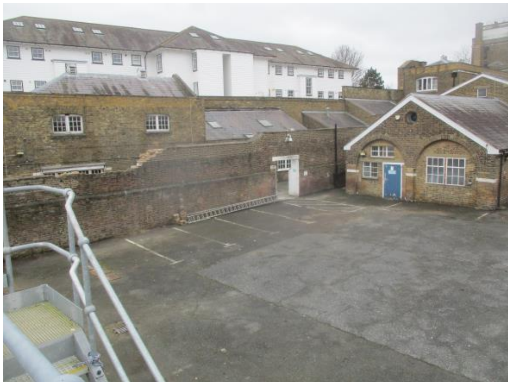
Plate 6. The boathouse with a walled walkway and adjacent workshops and offices to the east (looking south east)
