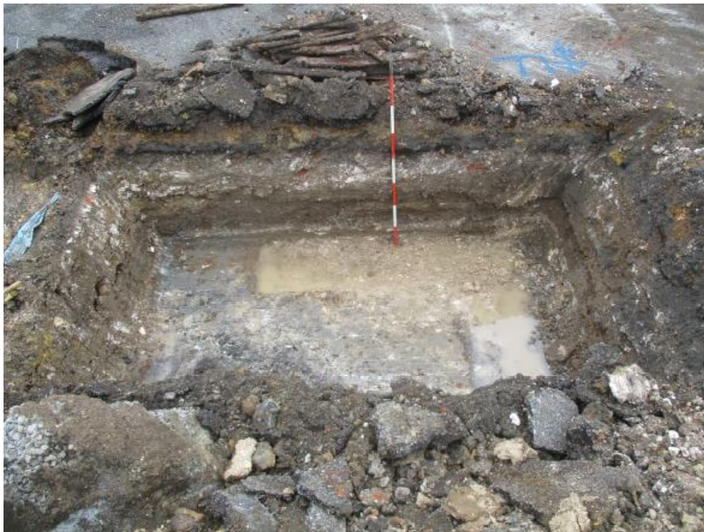
Plate 12. Trench 1. As above showing a pile of rusted steel objects comprising part of the channel's backfill (1.4m scale), from deposit 108
