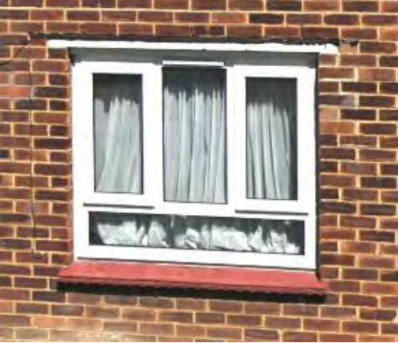
White window with timber header and red feature cil.
