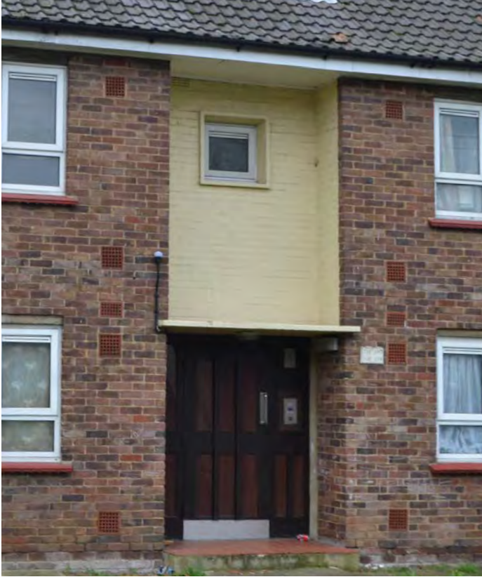
Recesses to communal entrances highlighted with painted brick
