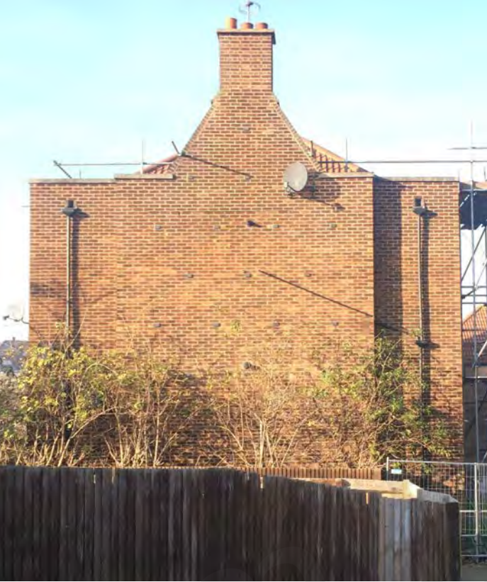
Stone capped gable with chimney with several interesting features including: Stepped Brick, English Bond, extruded brick patterning and brick capping detail.
