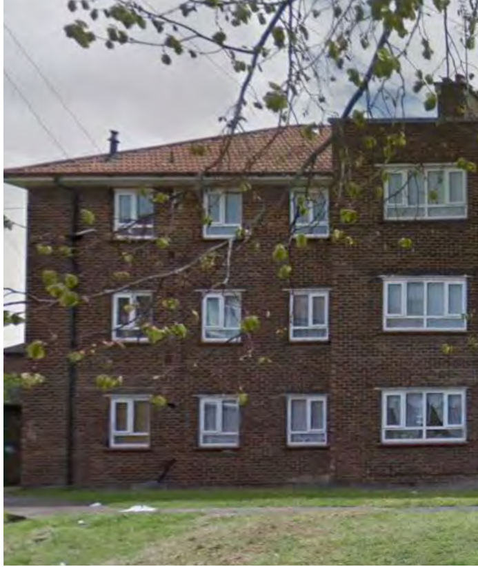
The existing buildings consist of a simple facade treatment, with ordered window arrangement, single material treatment and pitched roof consisting of red roof tiles.
