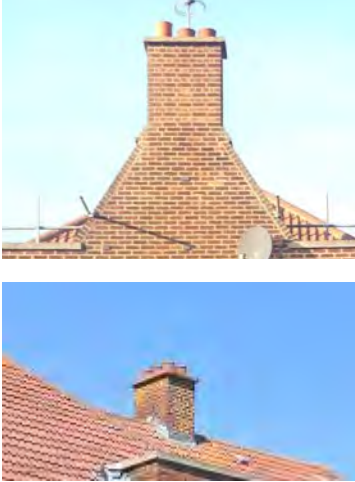
Feature chimneys contribute to the symmetry of the building.
