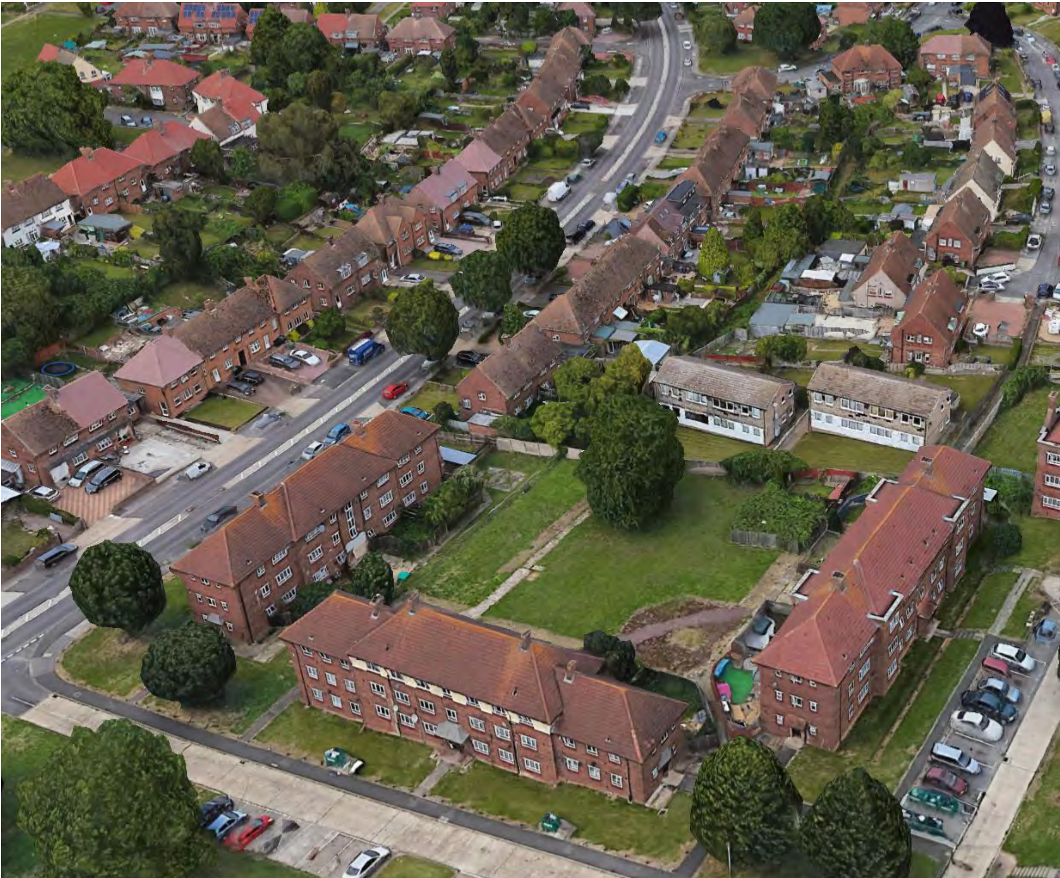
Aerial view of existing site
