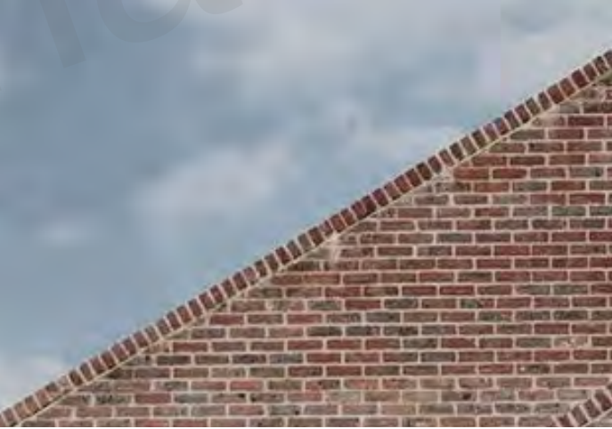
Brick rowlock capping detail
