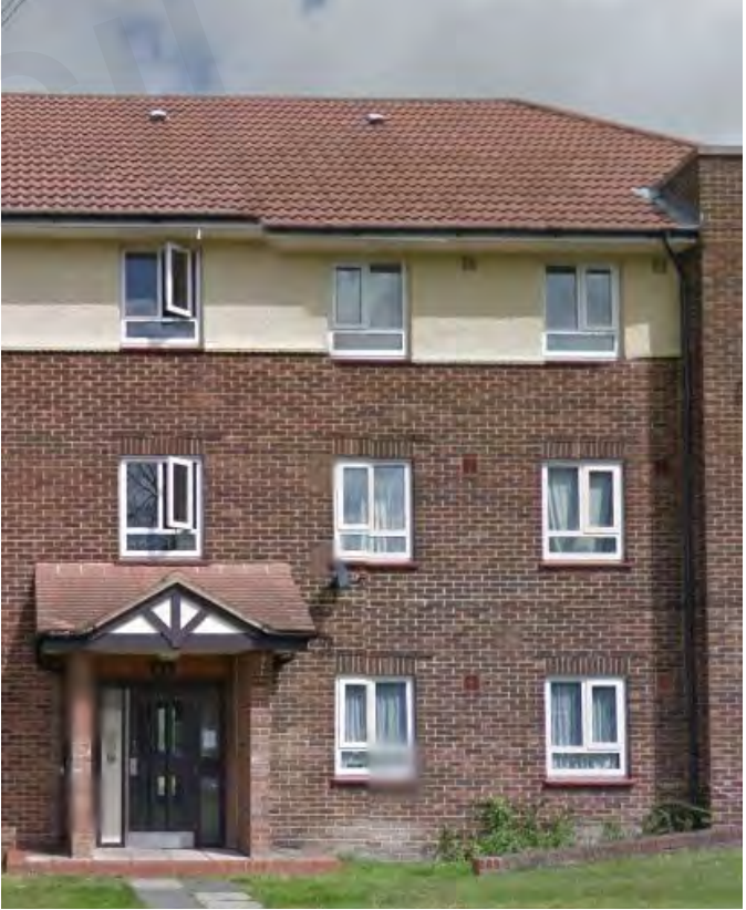
Brick banding and render upper floor contributes to providing a clear facade hierarchy.
