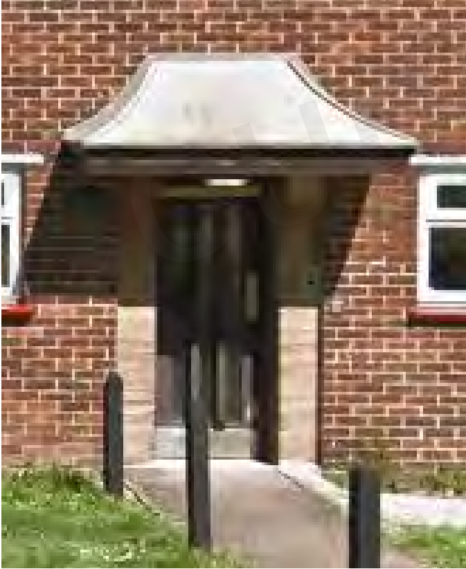
Tile creasing and canopy to communal entrance.
