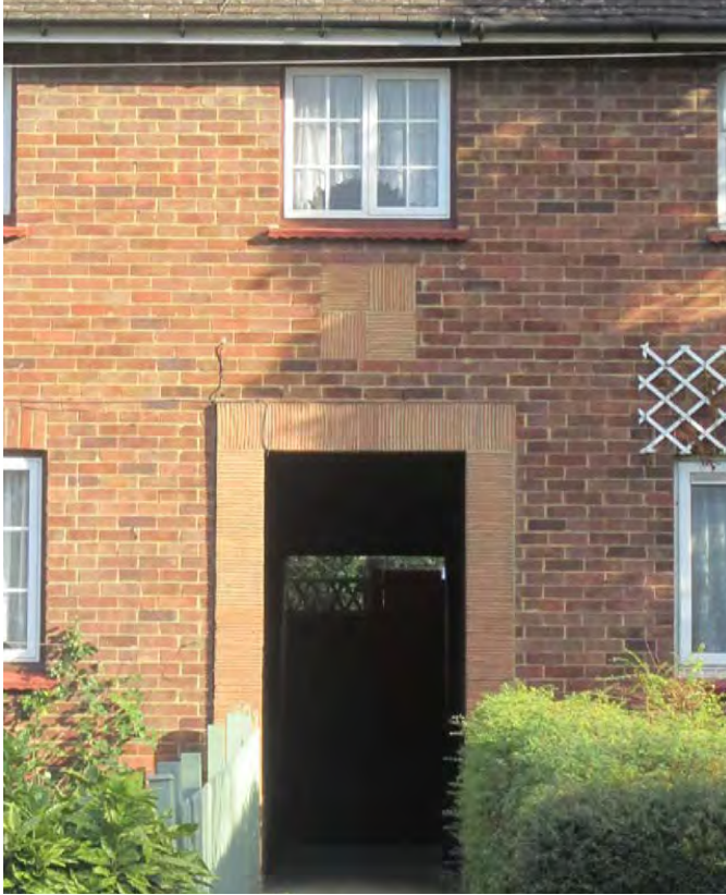
Projected creasing tile communal entrance surround and basket weave head decoration.
