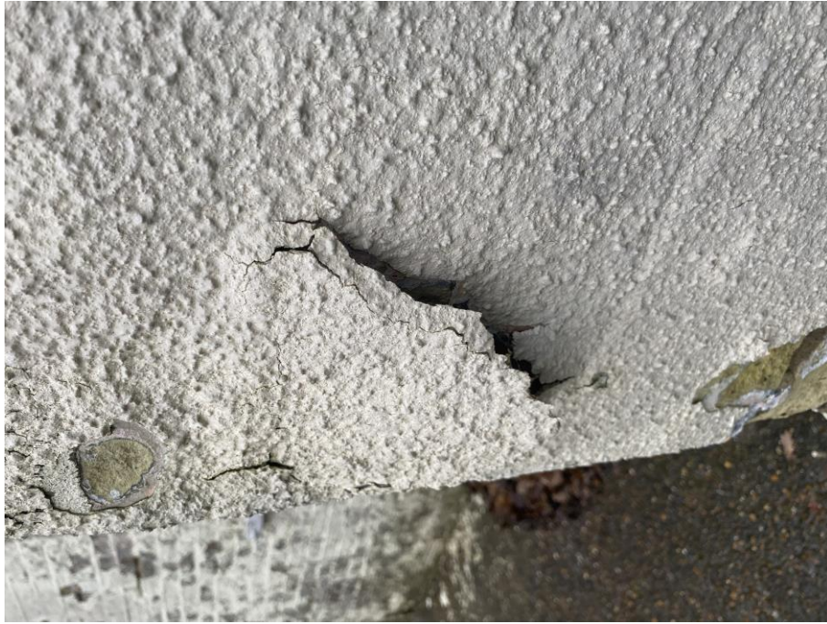
TEXTURED FINISH APPLIED TO BRICKWORK ON FRONT ELEVATION
