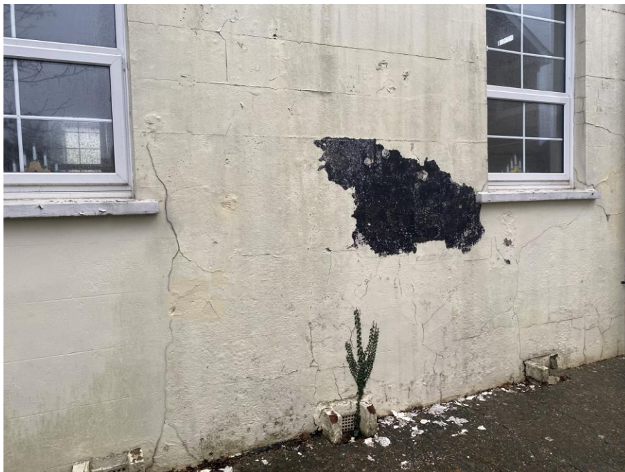
SIDE (SOUTH) ELEVATION – SAND/CEMENT RENDER FINISH
