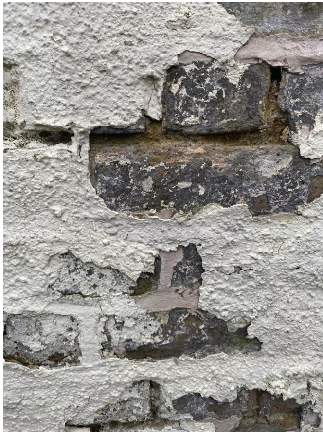
TEXTURED FINISH APPLIED TO BRICKWORK ON FRONT ELEVATION
