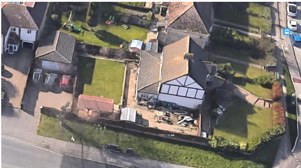
Fig 009 Aerial view of site looking west
