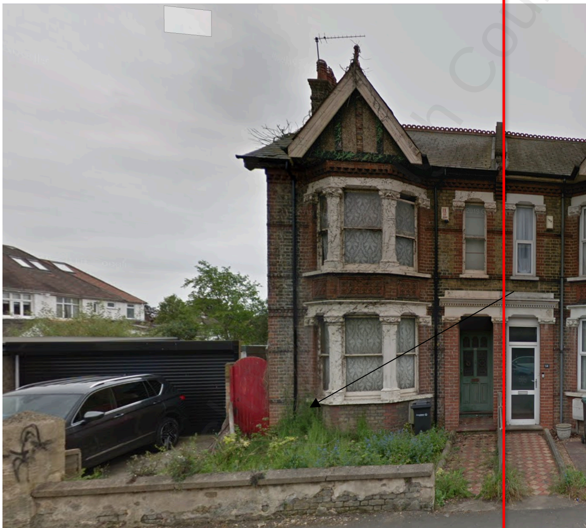
Photo showing 16 Lennox Road East front elevation
