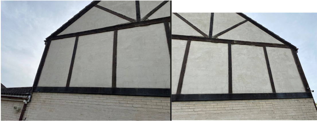
Fig 014 east gable wall detailing
