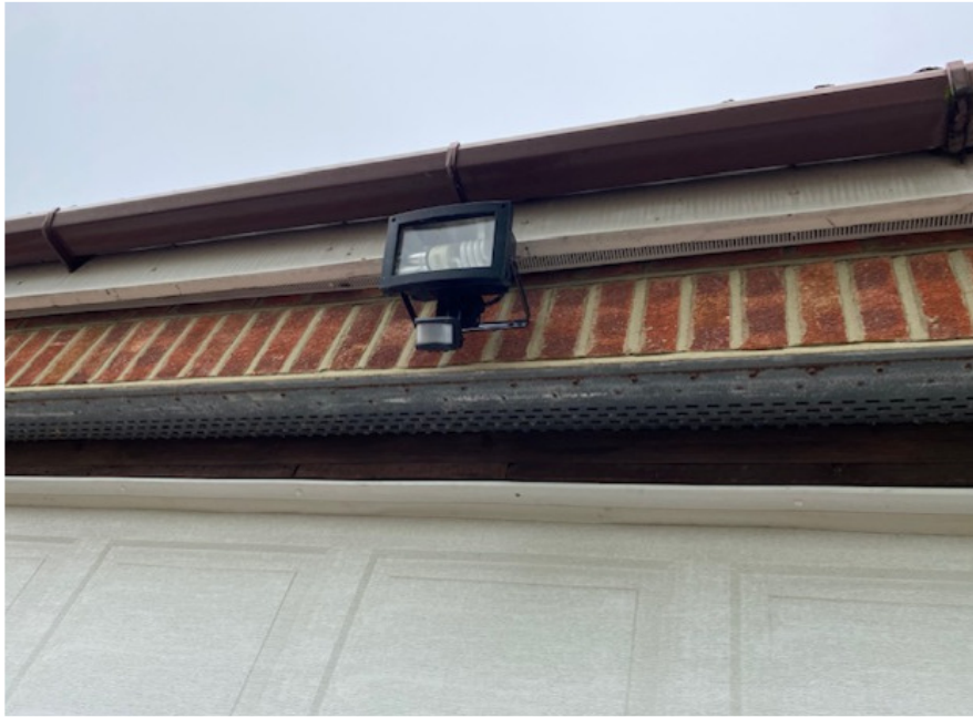
Fig 002 rear garage eaves
