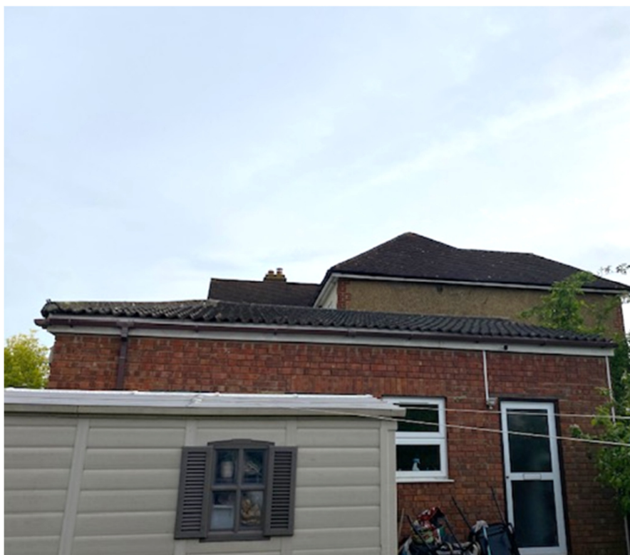
Fig 009 garage elevation facing main property
