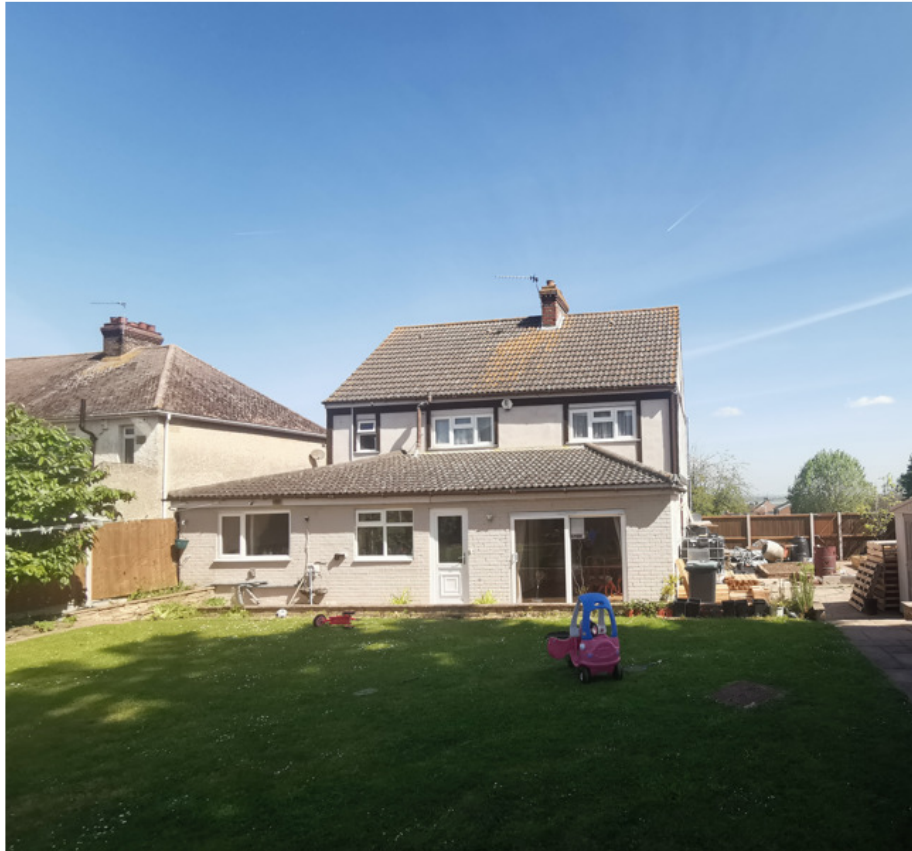
Fig 016 rear garden looking northerly back to main house
