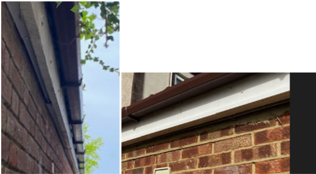
Fig 018 rear extension to main house soffit detailing.
