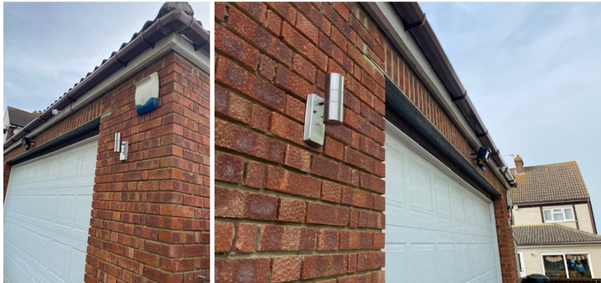
Fig 003 rear garage eaves details indicating soffit trim
