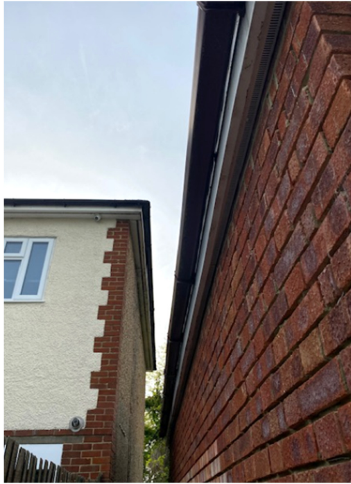
Fig 005 garage elevation adjacent to neighbouring property
