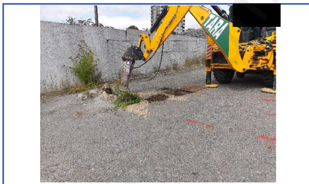
Manhole cover west of the subject site
