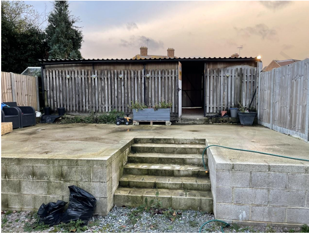
P01 – View showing the existing garage and upper level of rear garden
