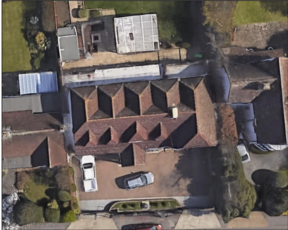
Figure 3: A large roof area at 234 Singlewell Road, next door to the application site.
