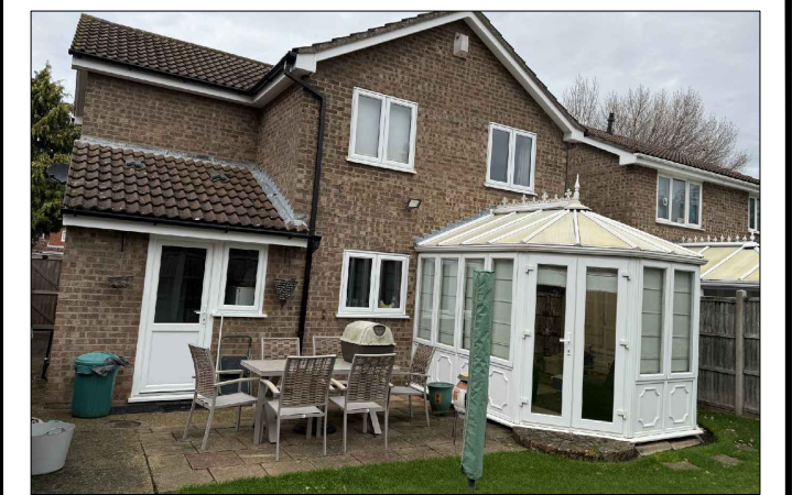
Photo Of Rear Elevation
