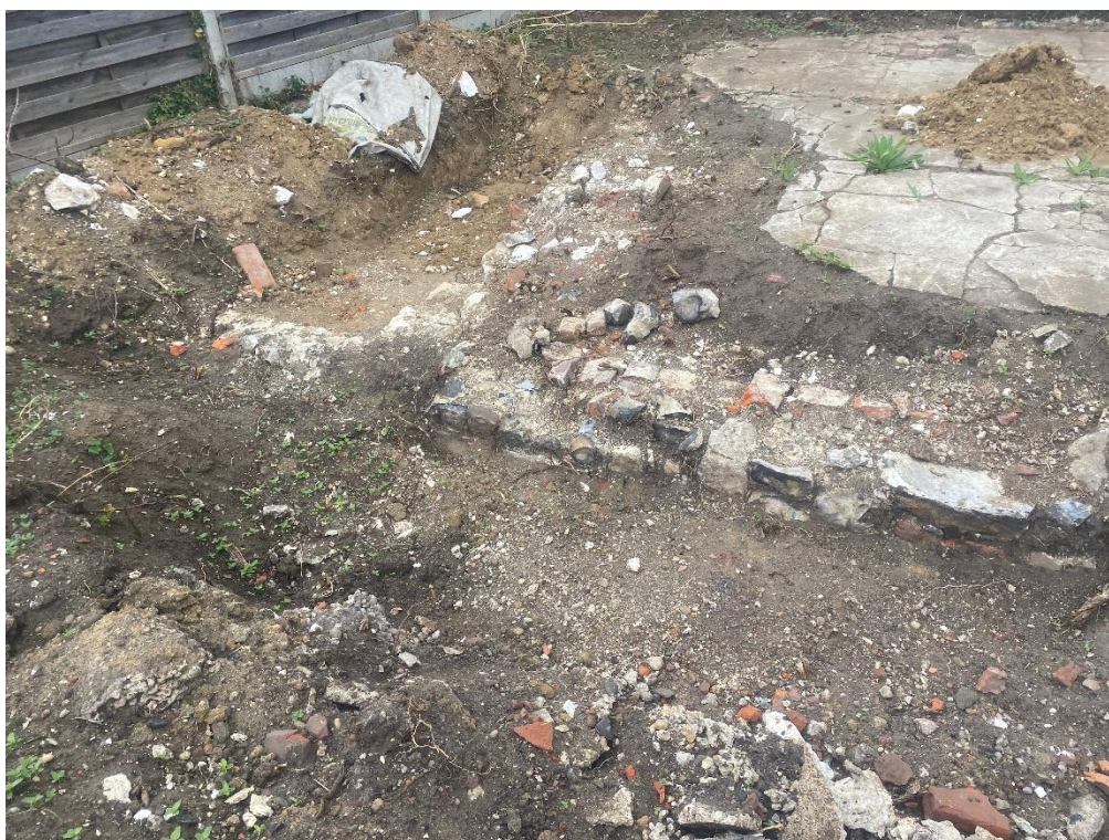
Figure 5.6 Image of previous foundations evident on site
