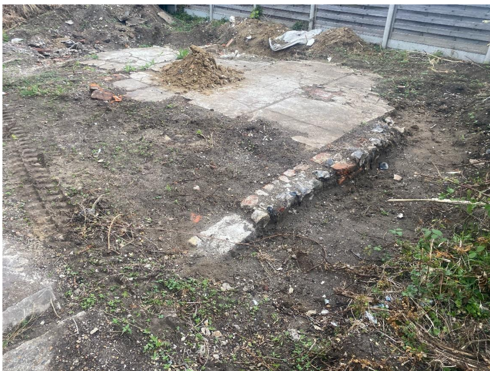
Figure 5.4 Image of previous foundations evident on site
