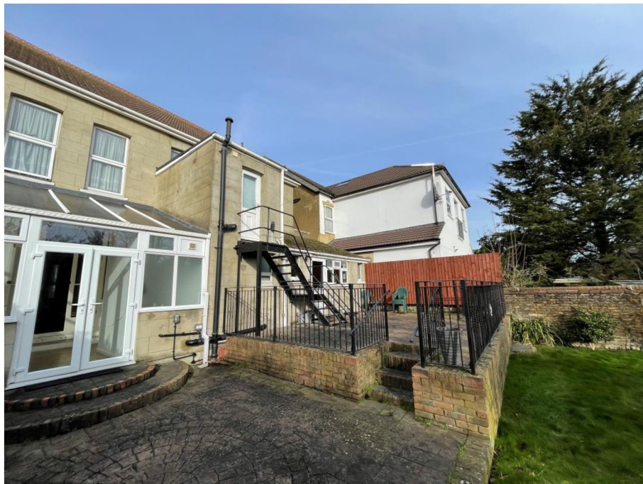
Fig 3 – Rear of No.54 Pelham Road
