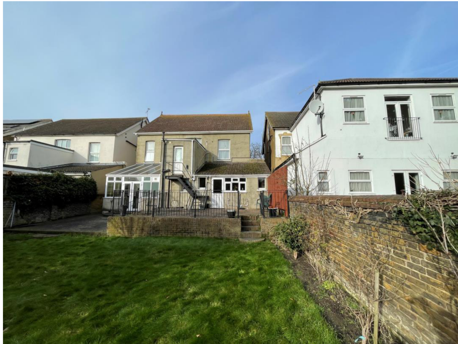
Fig 2 – Rear of No.54 Pelham Road
