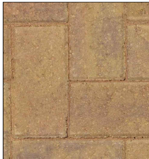
Path to Flat Entrances Marshalls Keybloc pavers Colour - Bracken
