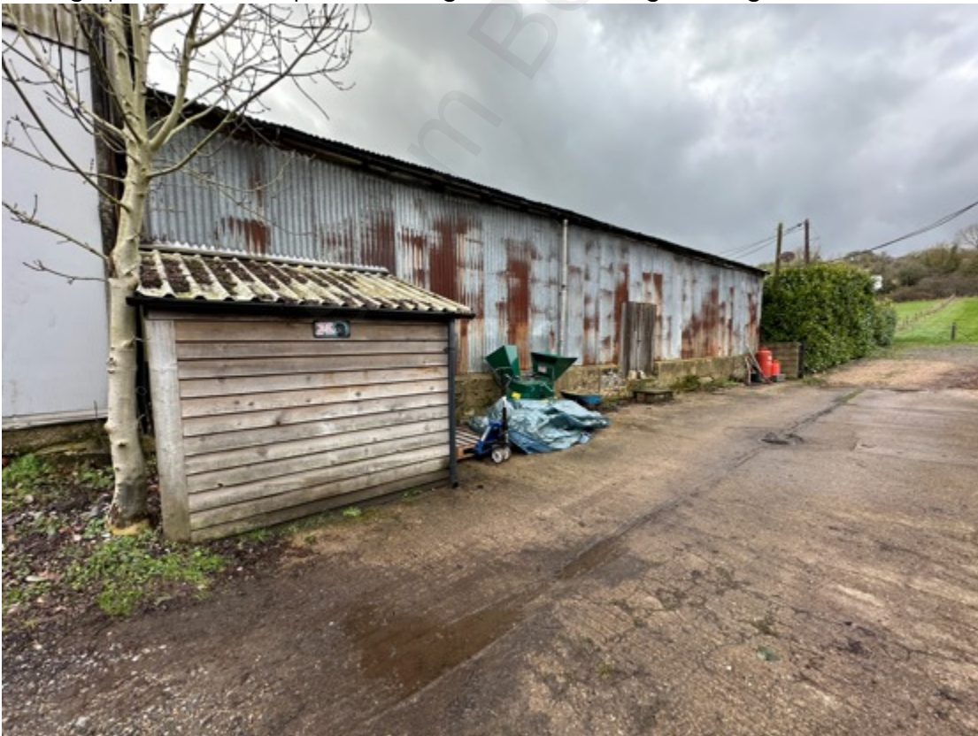
Photograph 6: Eastern aspect of the agricultural building, looking north
