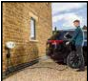
Car Charging Point in Car Port
