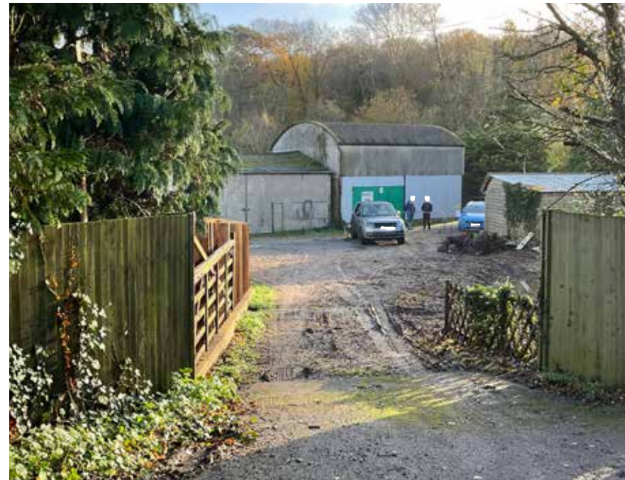
Image of entrance to the site
