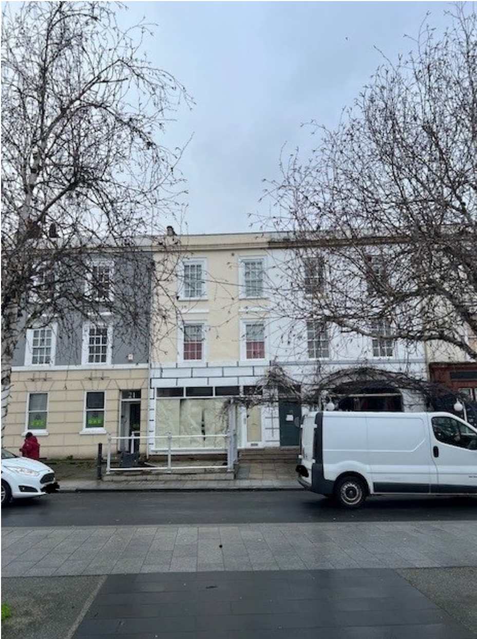
No. 22 Stone Street (the building with white painted ground floor shopfront & beige painted upper floors)
