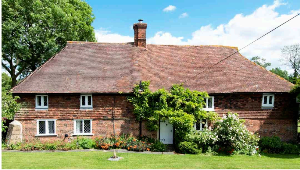
west elevation of house
