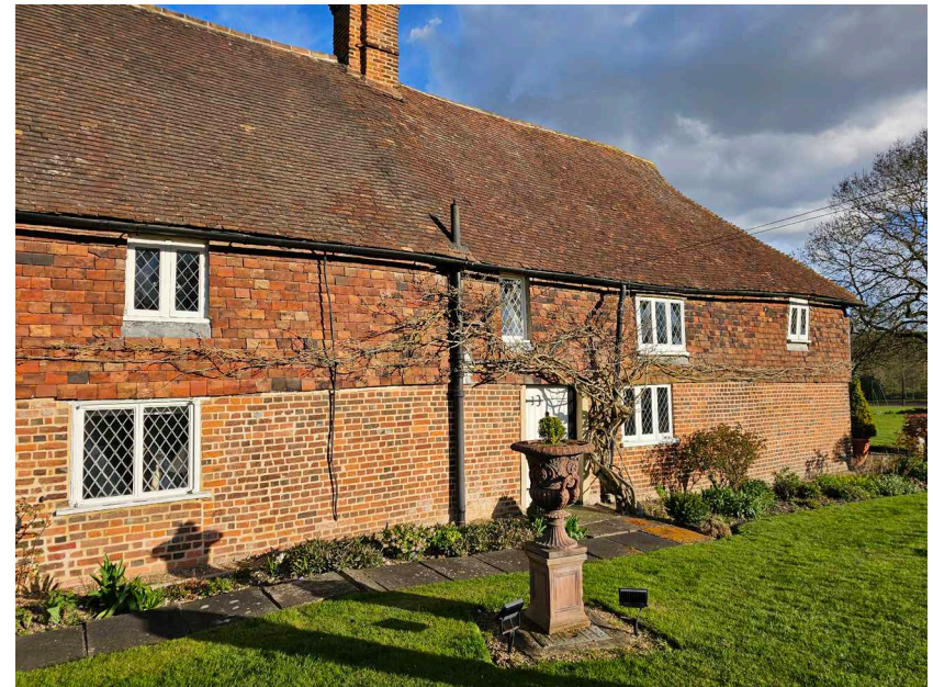
west elevation of house
