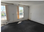
2nd Floor front room
