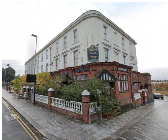
View from north-east on corner of Stone Street and Athboy Road
