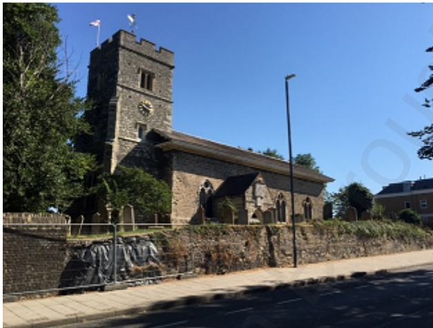
Flint section of the wall along East Milton Road, including the collapsed section
