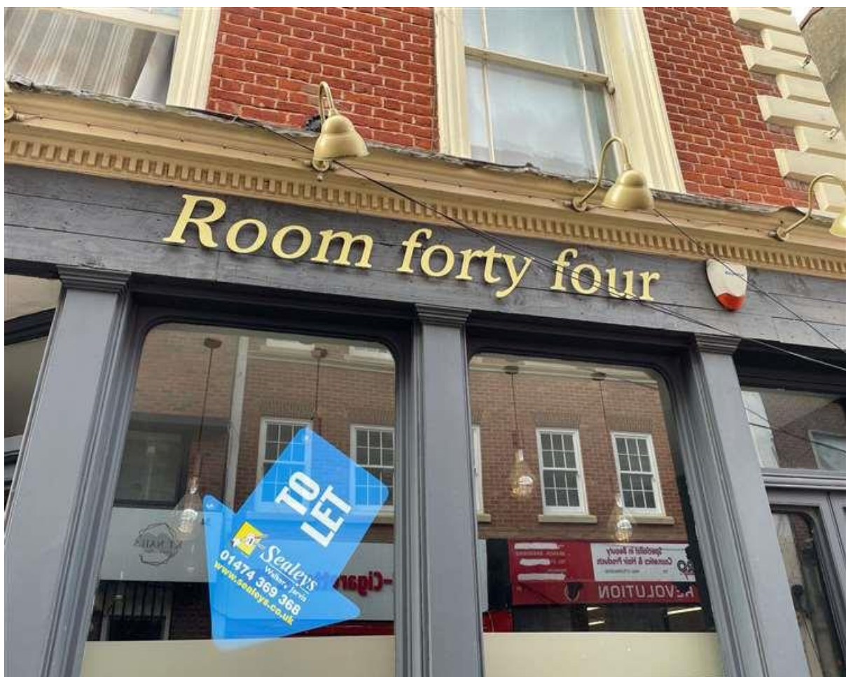
Existing Shop Front- Room Forty Four
