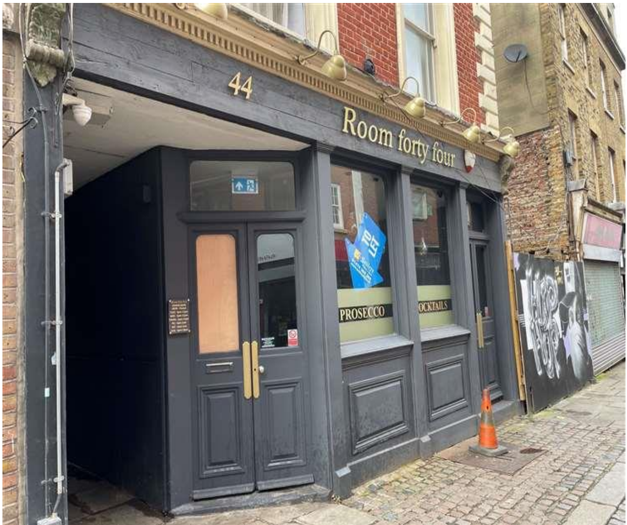
Existing Shop Front- Full View
