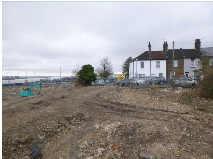
Photograph 4: Showing the site and further cleared ground to the north
