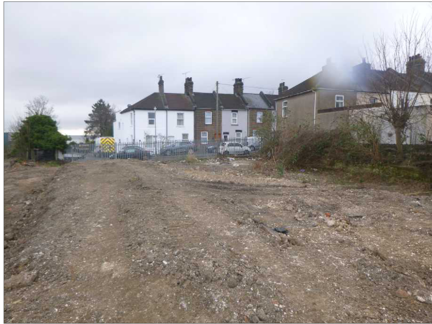
Photograph 1: Showing the site facing east.
