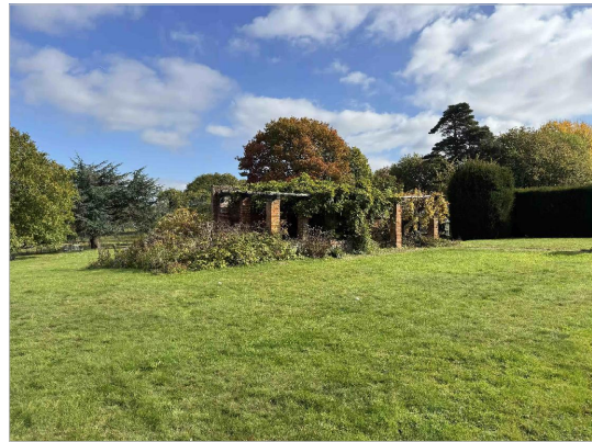
1. LOGGIA EXISTING PHOTOGRAPHS
