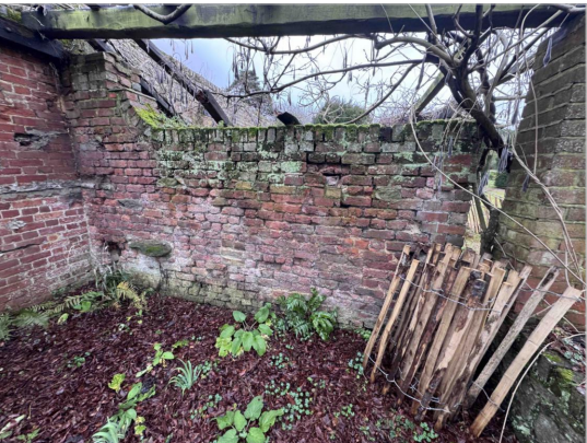
2. VIEW OF CENTRAL BRICK DIVIDING WALL
