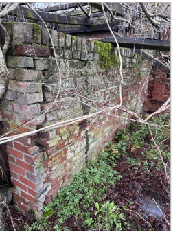
3. VIEW OF OTHER SIDE OF CENTRAL BRICK DIVIDING WALL ( LIMITED ACCESS)
