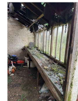
6. INTERNAL VIEW SHOWING WORK BENCH & EXPOSED STRUCTURE
