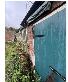
3. STORAGE OF ROOF TILES TO BE REPLACED
