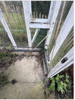
4. CONCRETE FLOOR SHOWING BRICK PLINTH WITH LEADED CILL
