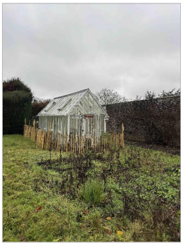
1. VIEW OF GREENHOUSE FROM EAST
