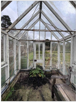
3. INTERNAL VIEW LOOKING EAST
