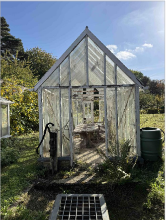
7. VIEW OF SOUTH WEST ELEVATION
