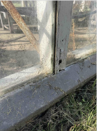
8. CLOSE UP OF LEADED BRICK PLINTH AND ROTTEN TIMBER WALL PLATE
