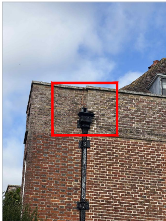
2. VIEW OF THE DRAINAGE OUTLET, HOPPER AND DOWNPIPE
