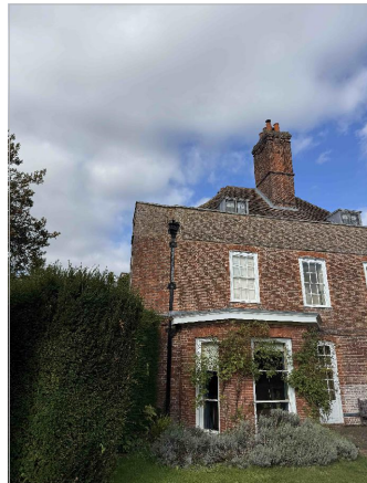
1. VIEW OF SOUTH EAST ELEVATION
