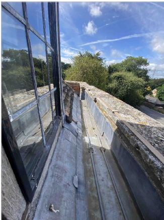
4. LEADED STEPPED GUTTERING BEHIND THE PARAPET WALL
