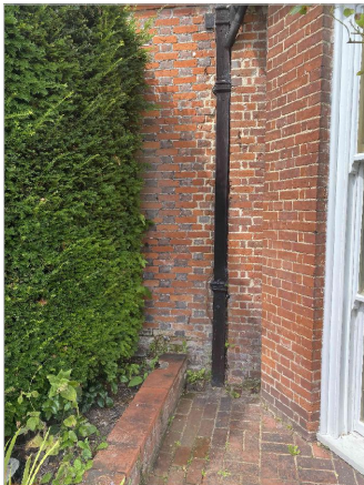
3. GULLY WHERE THE DOWNPIPE DISCHARGES
