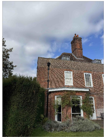
1. VIEW OF SOUTH EAST ELEVATION
