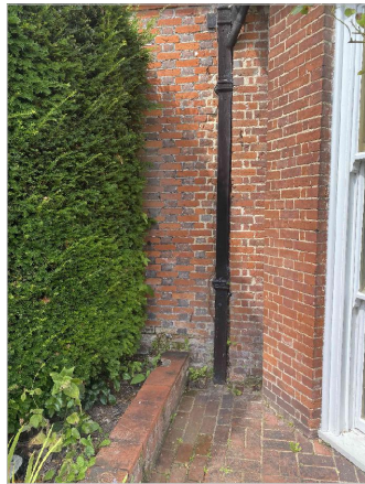
3. GULLY WHERE THE DOWNPIPE DISCHARGES
