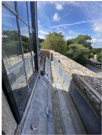
4. LEADED STEPPED GUTTERING BEHIND THE PARAPET WALL
