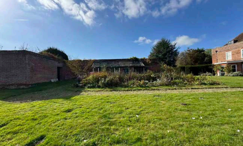
3. View of Potting Shed structure
