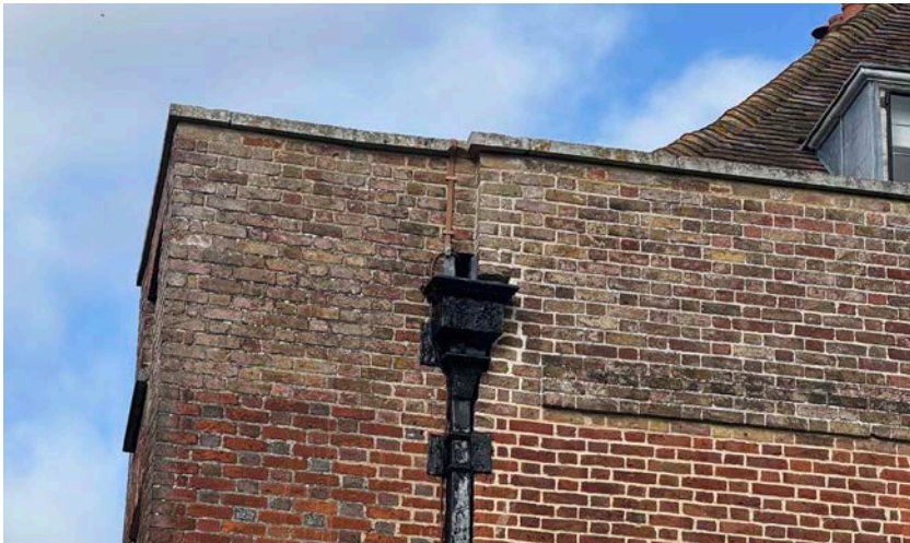
2. Close up of gutter outlet, hopper and downpipe
