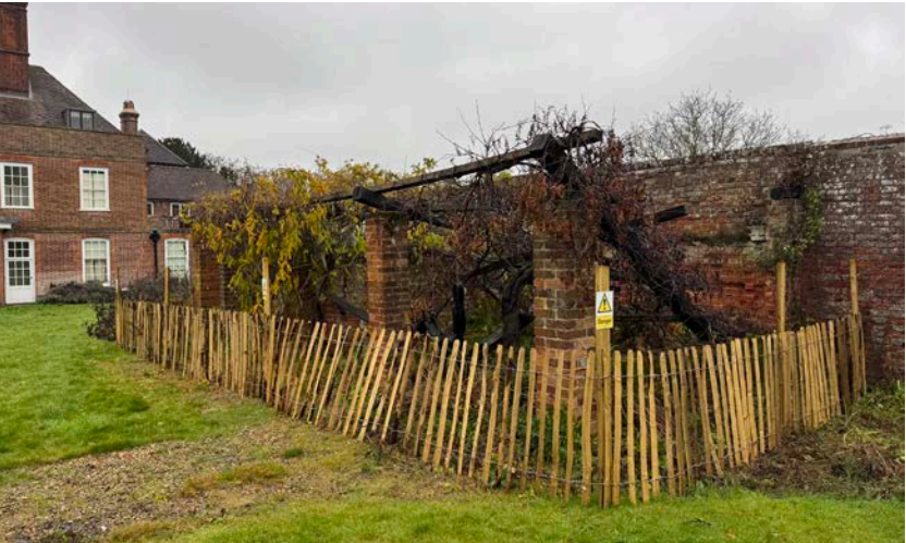
1. View of Loggia from south with Owletts Mansion behind
