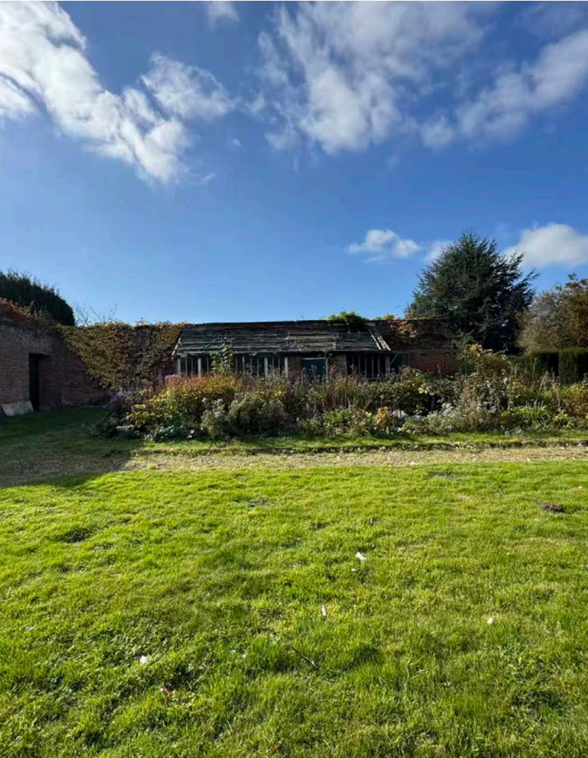
1. North elevation of potting shed
