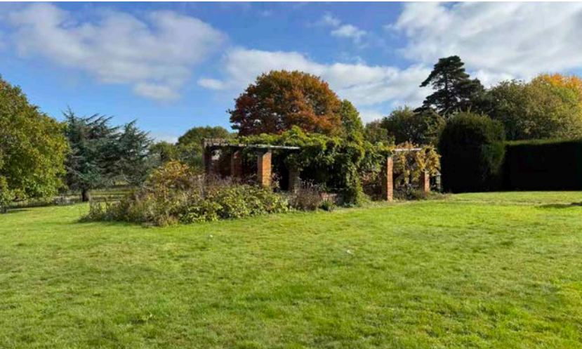
2. View of Loggia structure
