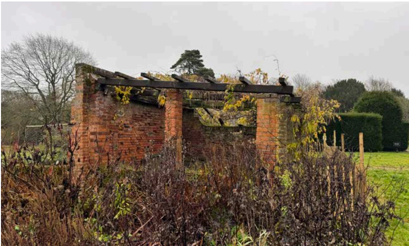
2. View of north west elevation of Loggia
