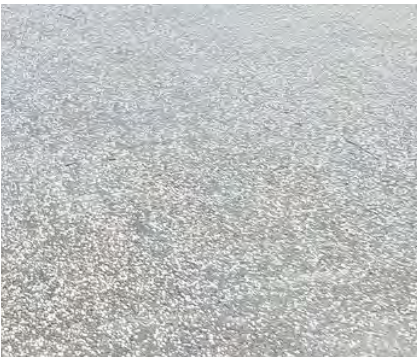
In situ exposed grey aggregate poured concrete
