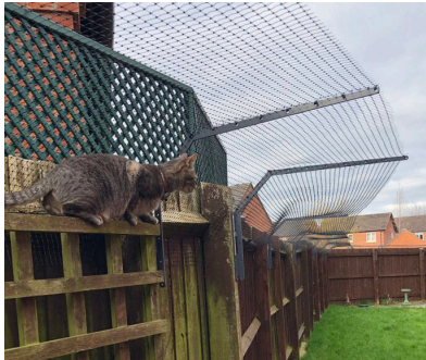
Provision of cat-proof fencing at the boundary adjacent to the SSSI
