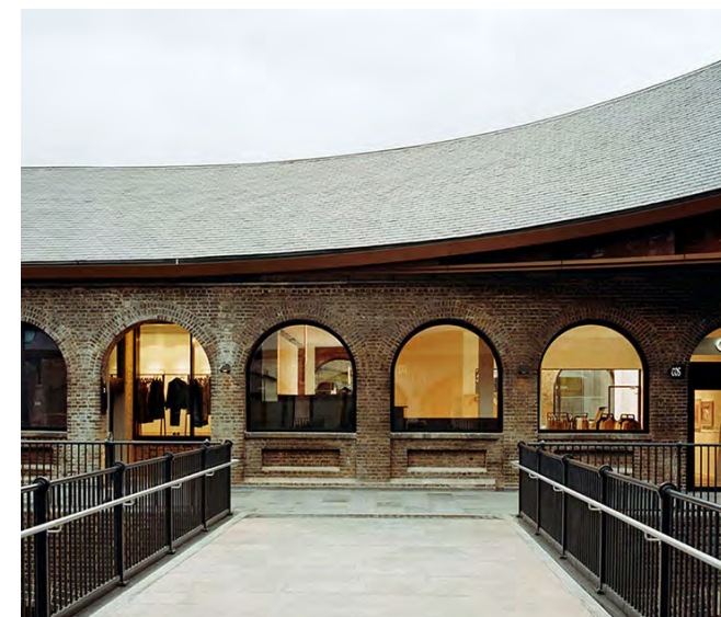
Coal Drops Yard - Heatherwick Studio
