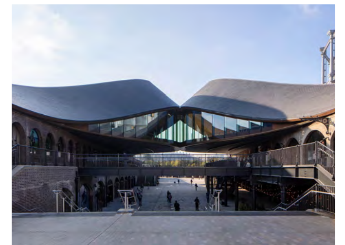
Coal Drops Yard - Heatherwick Studio
