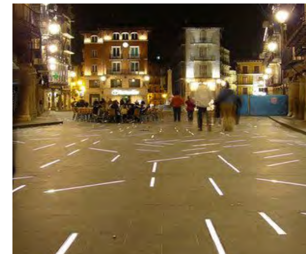
Lighting incorporated into paving
