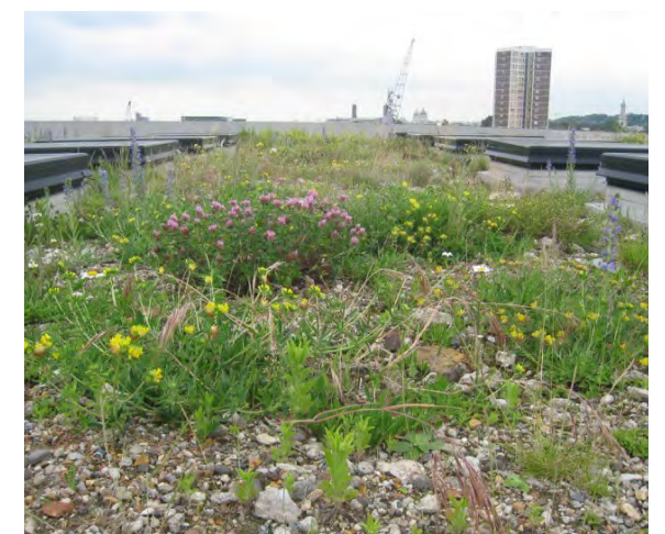
Planted green/brown roofs
