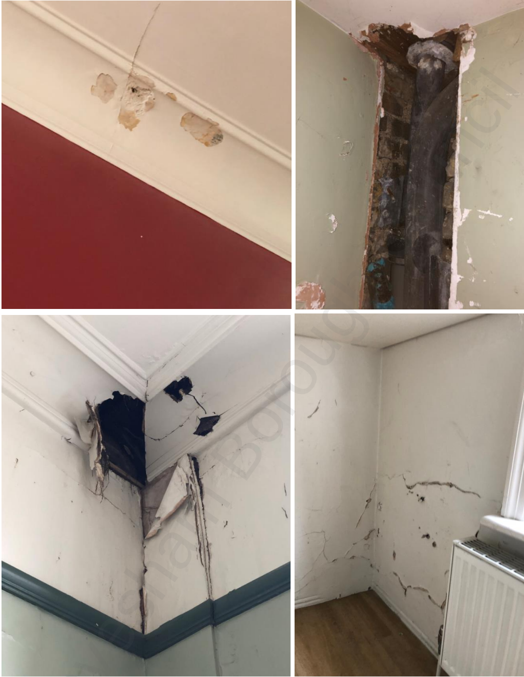
Figure 10 – Plaster and rainwater pipe repairs
