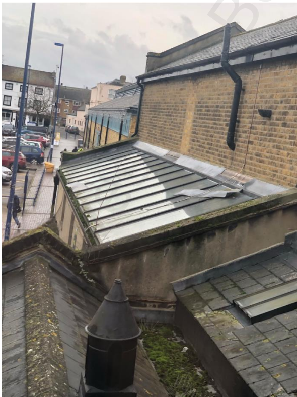
Figure 2 – Down Pipes and gutters
