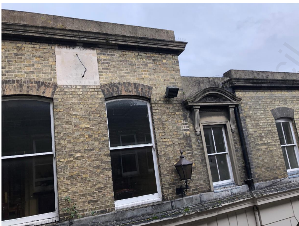
Figure 3 – Stone and Render repair
