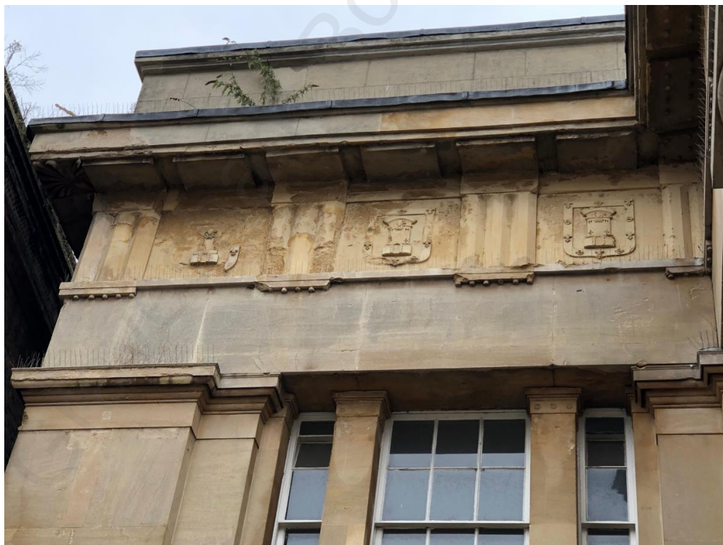
Figure 4 – Stone repair – LHS of portico at main front entrance Gravesham coat of arms detail eroded
