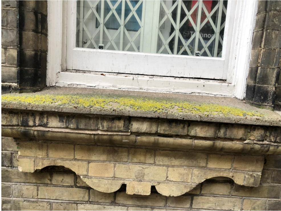
Figure 7 – Window repair and repaint
