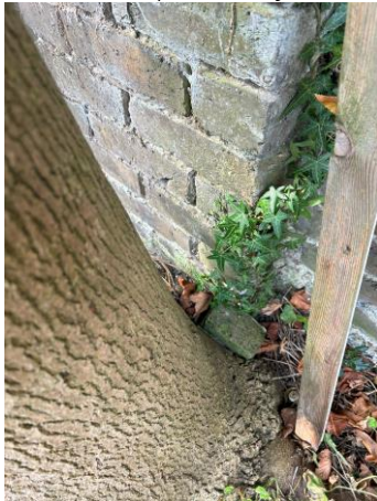
Pic. 7 Wall proximity T1
