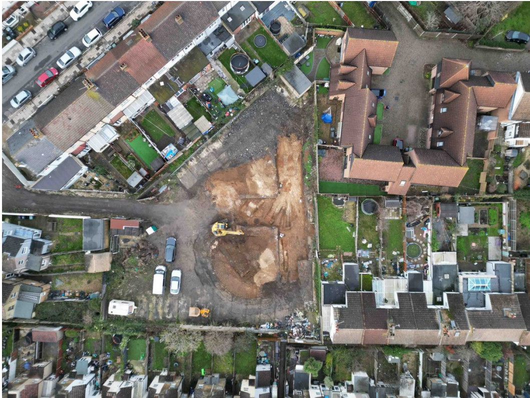
Plate 7: Drone site view; north to the top
