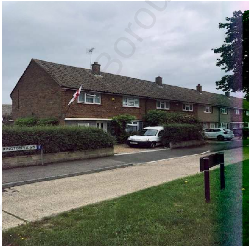
Photograph Showing the Front View of Land
