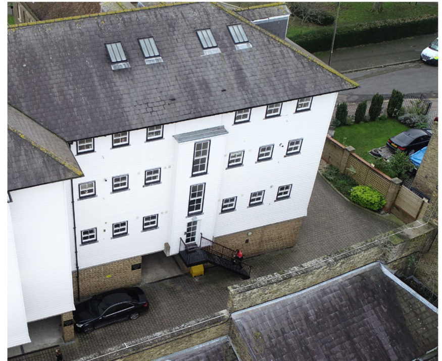
Image 4 – External aerial drone image showing the windows in Heritage Quay
