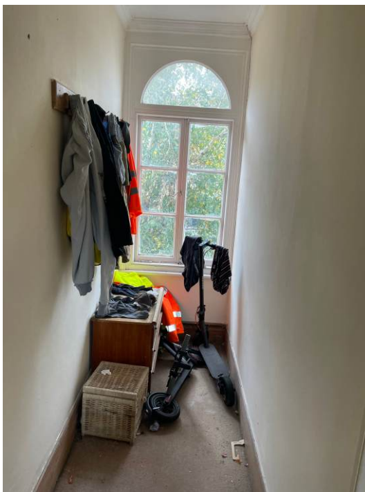
PHOTOGRAPH 6 Landing window at first being an intact original photograph it also illustrates the existing skirtings which are generally intact throughout
