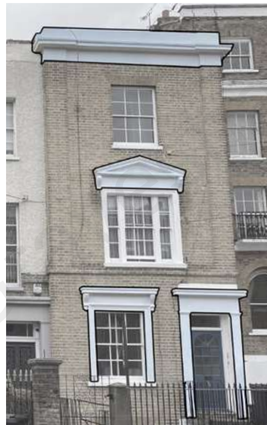
Decorative banding and moulding to parapet, window and door openings.
