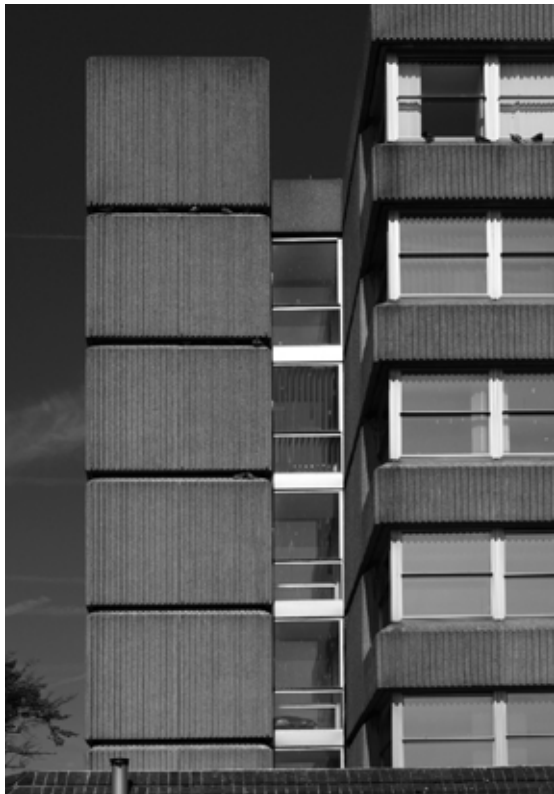
Detail bay of concrete facade
