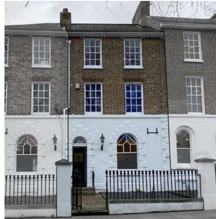
Dark buff brick work with white rendered ground floor. Georgian period windows, contrasting brick headers and fore-garden with black railing boundary.
