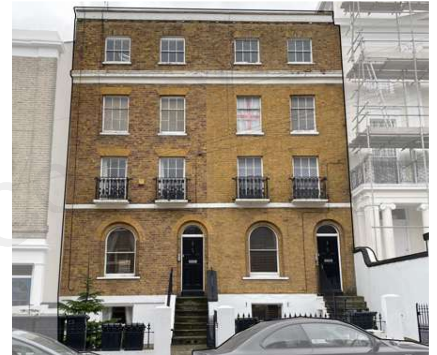
Five-storey terrace pair with contrasting buff brick. Decorative banding, splayed window headers, Juliette balcony and clear hierarchy of window proportions.
