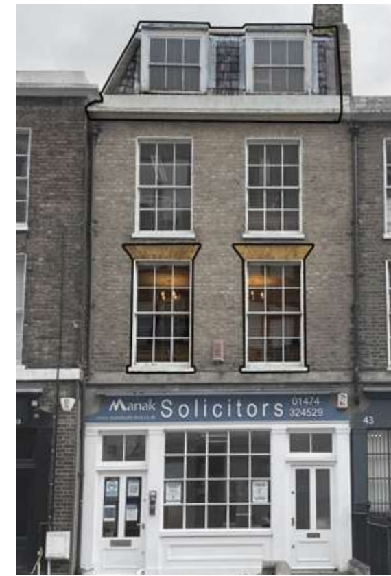
Splayed brick header in contrasting brick with dormer windows to slate mansard roof.
