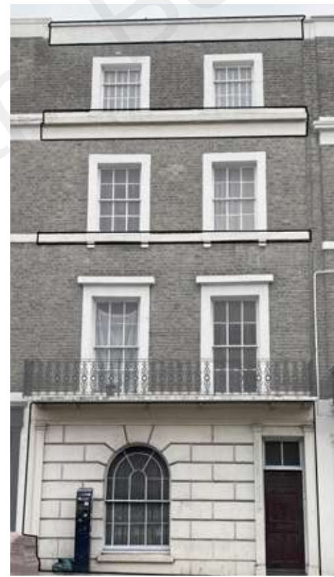
Decorative banding and rusticated render to ground floor.
