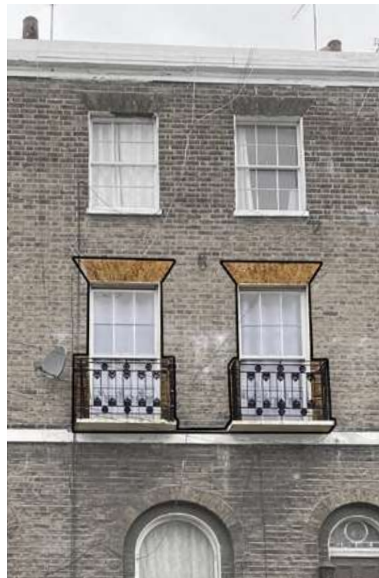
Georgian proportion windows with Juliette balcony and splayed window header.
