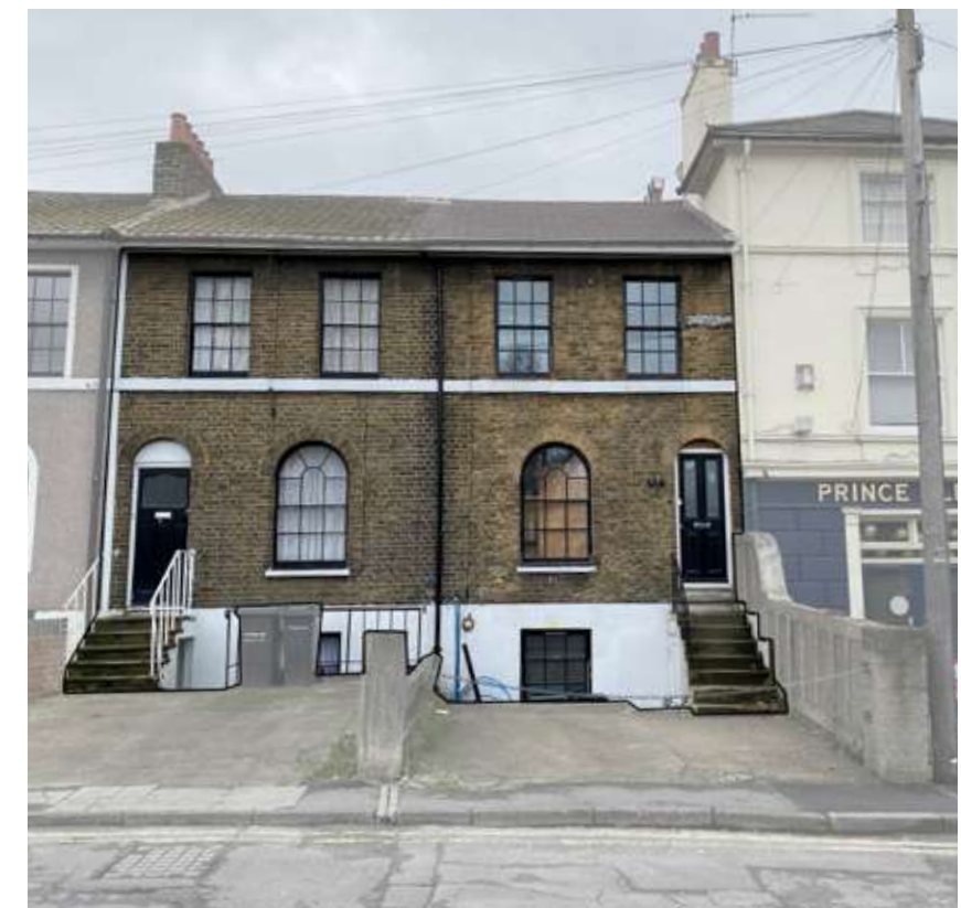
Pair of terraces characterised by contrasting buff / yellow brick stock with white rendered ground floor banding and solid front doors in traditional style.
