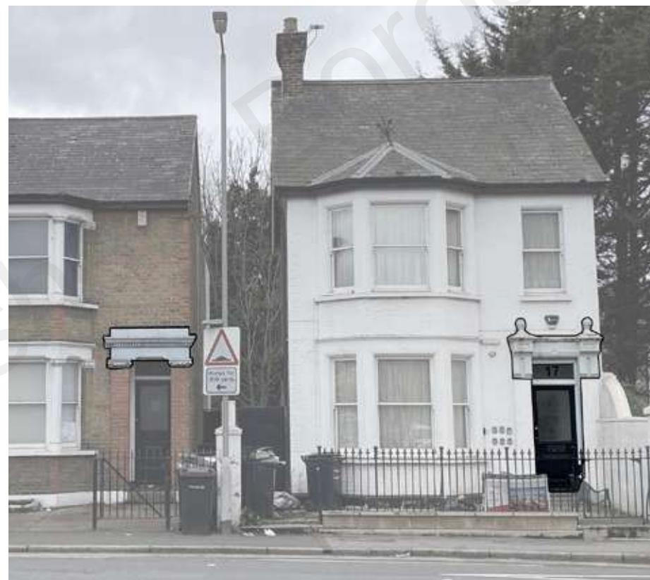
Decorative banding and moulding to window and door openings.
