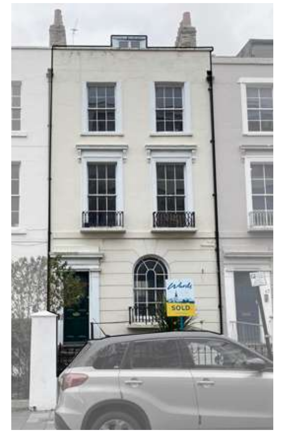
Rendered facade with rusticated ground floor section. Decorative moulding to window surrounds and Juliette balconies.
