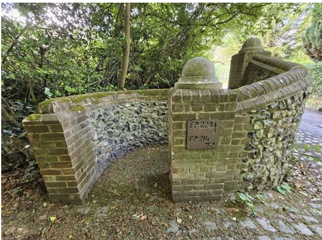
Fig.7: The northern (outer) opening is approximately one metre in width, flanked by modern brick piers.
