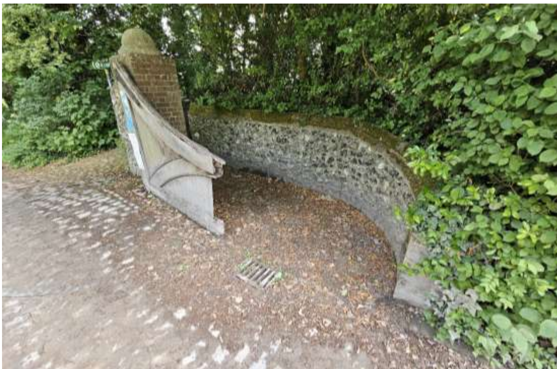
Fig.8: The southern (inner) opening is approximately 3.5 metres in width from pier to pier.
