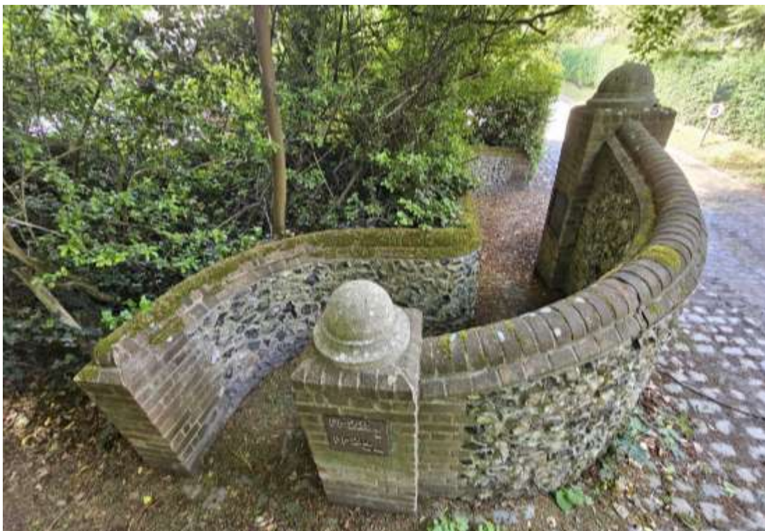
Fig.6: The curved layout of the walls and inner and outer access openings with the public path running between the two.
