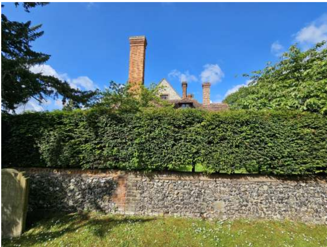
Fig.12: East elevation of Luddesdown Court seen over the wall and hedge boundary with the church. Note that the materials of the wall were used to inform the design of the application wall, though variation in condition marks a clear distinction in construction date.
