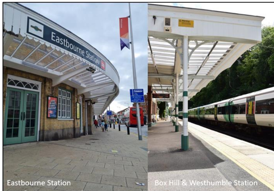
Figure 10: Examples of Plasiac glazing used at listed stations (Eastbourne and Box Hill & Westhumble)
