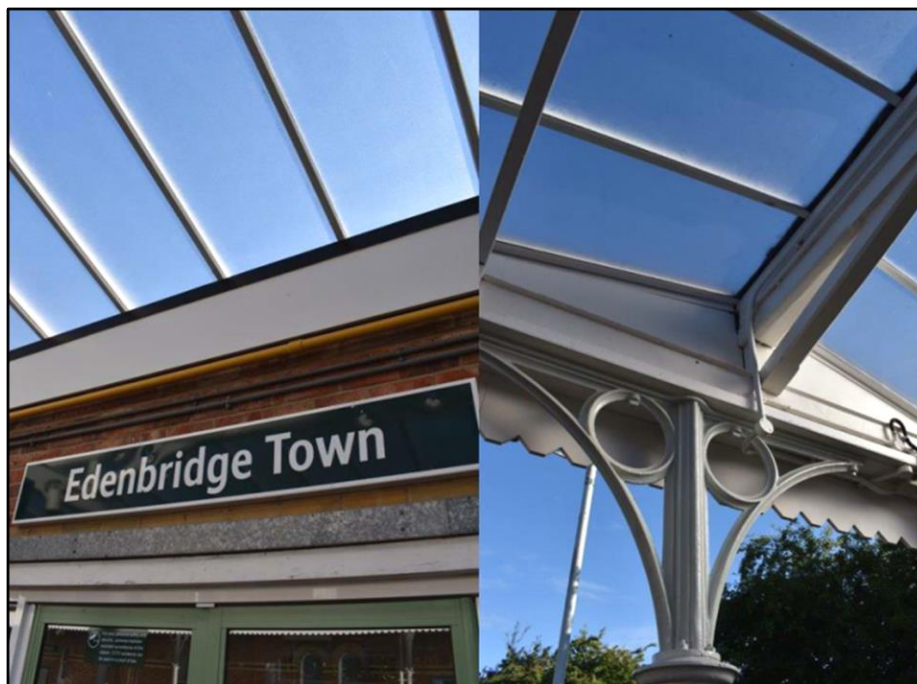
Figure 11: Obscured Plasiac glazing used at Edenbridge Town Station
