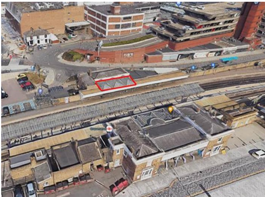
Figure 3: Area of glazing removed from Platform 2 canopy
