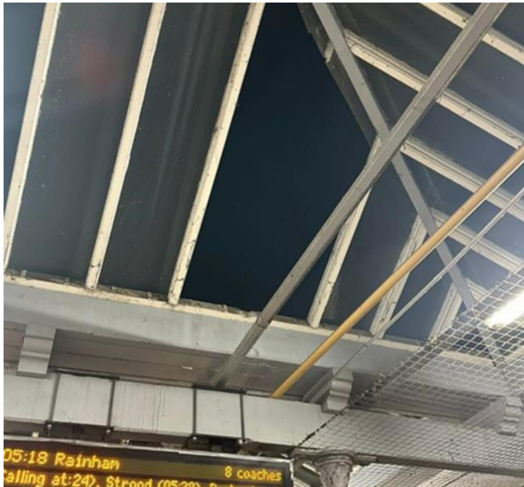
Figure 4: Underside of canopy showing routed edges to timber
