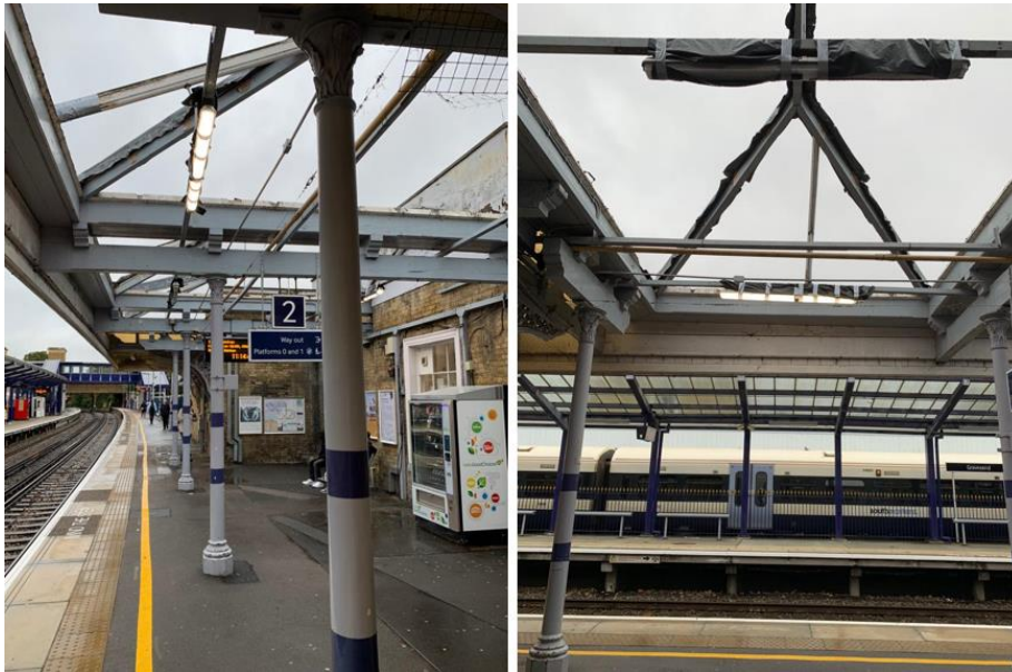
Figure 6: Exposed Platform 2 canopy
