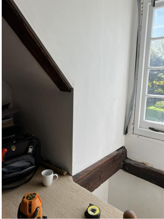
Image of existing dormer window, internally.
