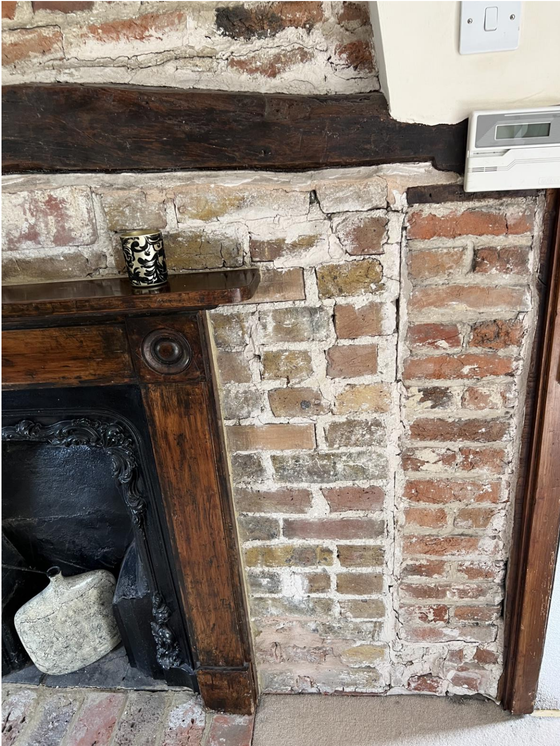
Image of the inserted fireplace and infill brickwork below the bressummer in the first floor of the axial chimney facing west.
