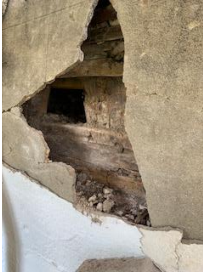
Inspection hole removing render build-up to expose framework behind.
