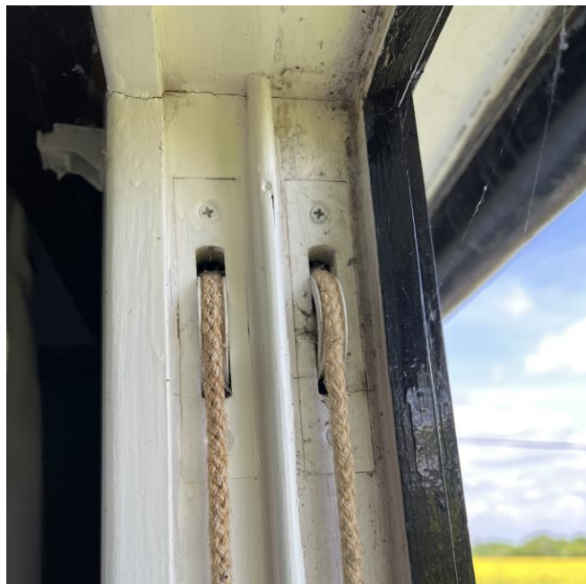
Internal image of the relatively modern axle pulley wheels and sash cords of the front elevation 'box-frames'.
