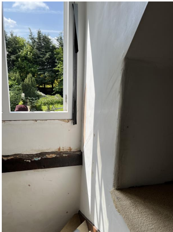
Image of existing dormer window, internally.
