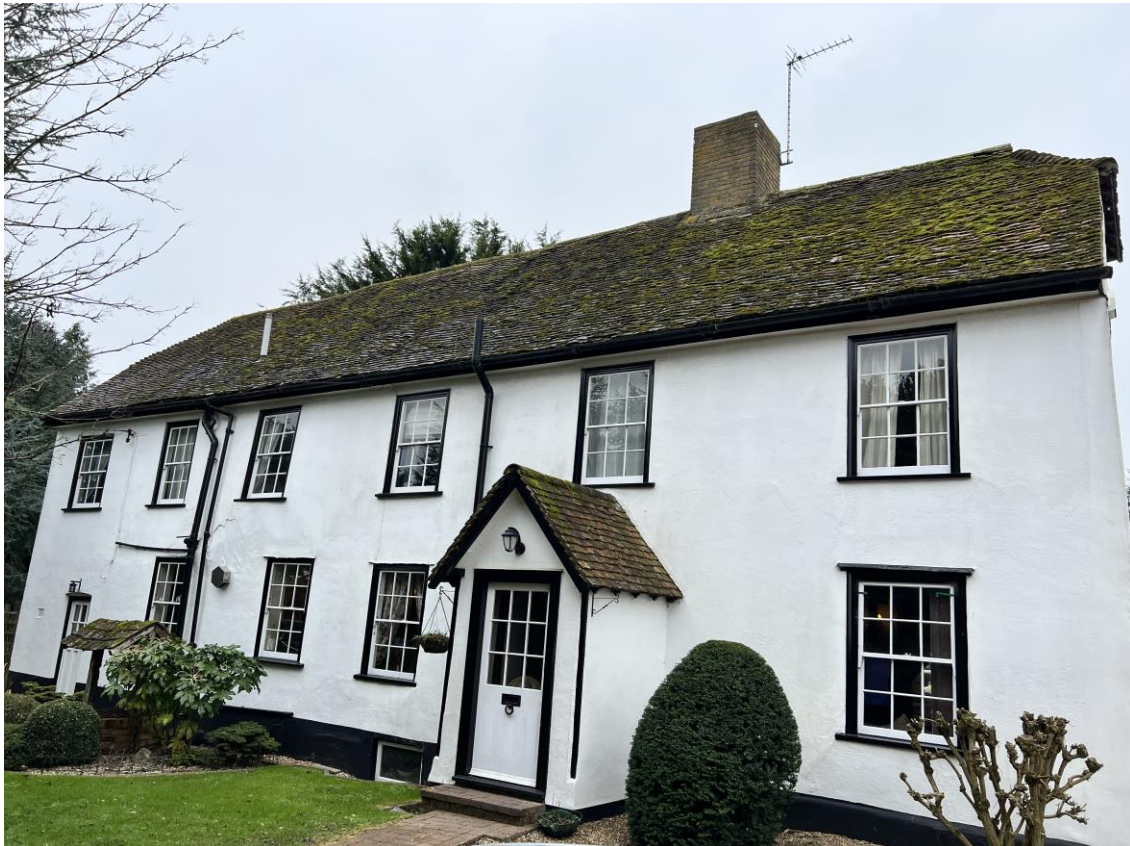
Image of the front (north) elevation.
