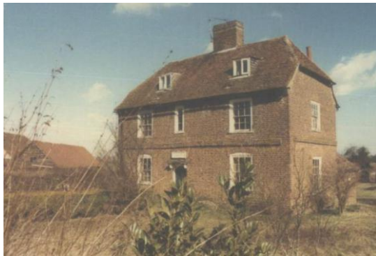
1982 photo of the SW & SE elevations
