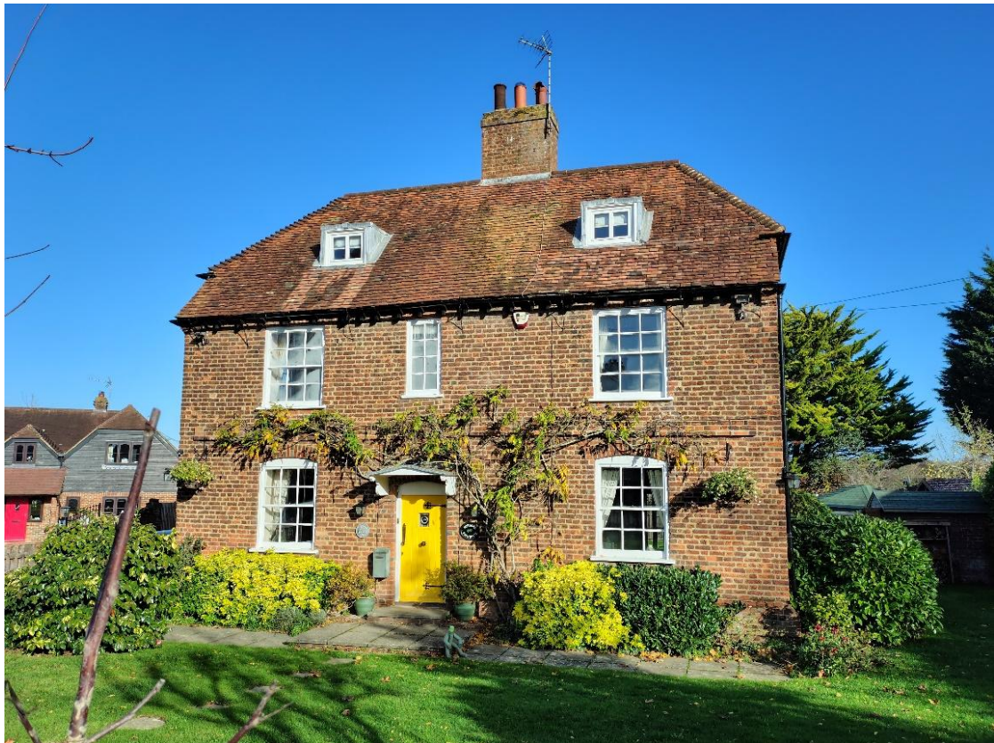
South-west (principal) elevation fronting Norwood Lane.
