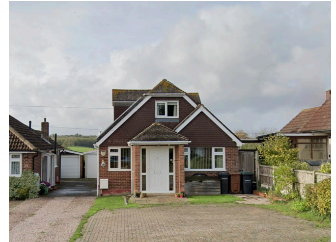
Fig.10 - Neighbouring property (No. 52) with red brick and tile
