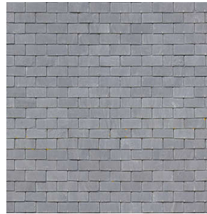
Slate Roof Tiles
