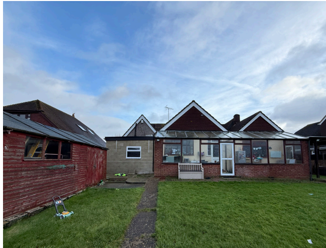
Fig.4 - Rear elevation of site showing existing extension
