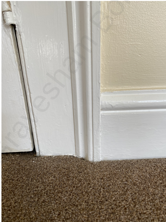
Second Floor Room 3
