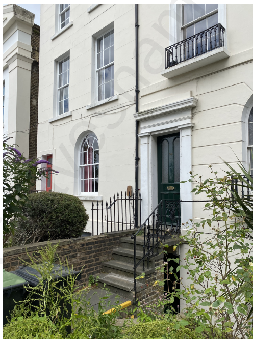
Metal railings at the front
