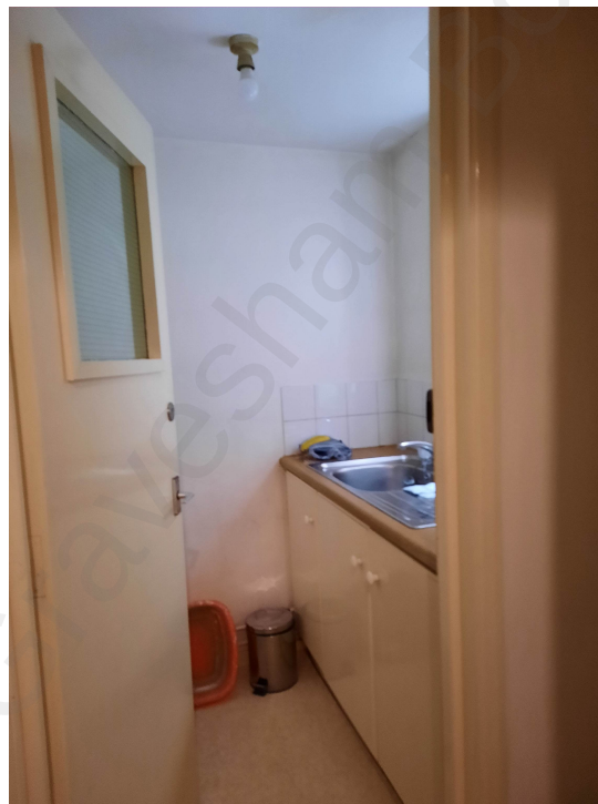
Rear Ground Floor Utility and WCs
